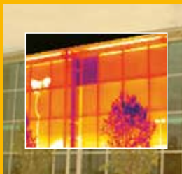
Thermal inspection of a window installation.
