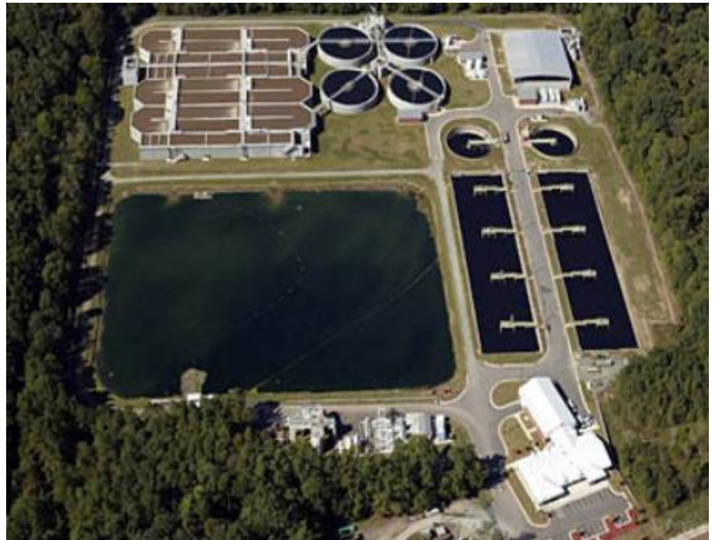
High-Tech treatment system
