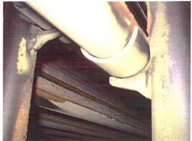
TYPICAL ARRANGEMENT OF SHIELDS FOR REAR WATERWALL HANGER TUBES
