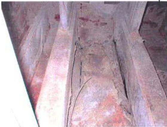
Actual in-field application of Isomembrane located just above the fire box.
