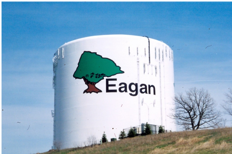
A Ground Storage Tank
