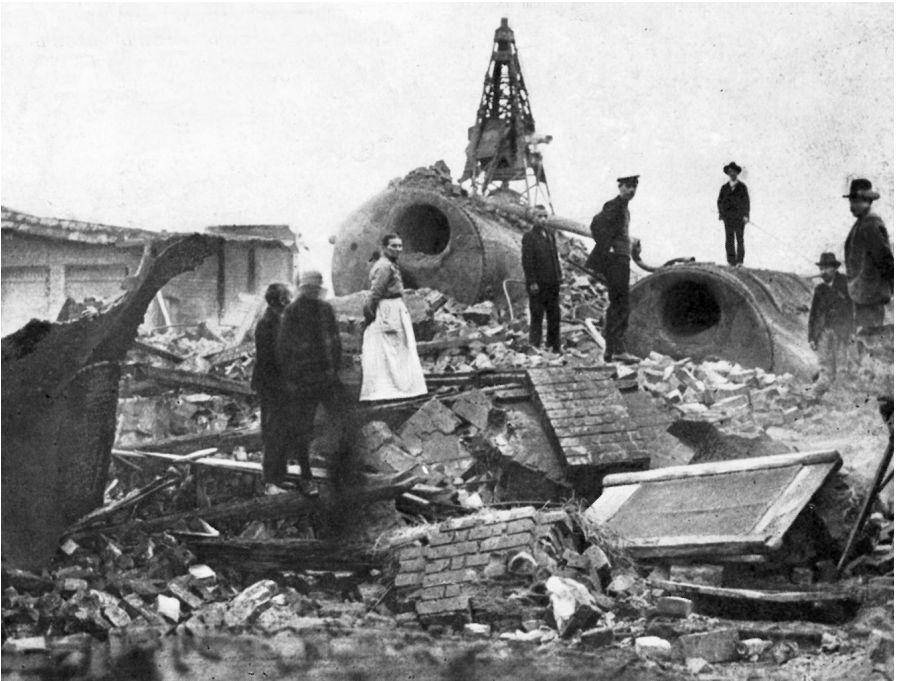
Figure 23: Destroyed factory building caused by a boiler explosion (Meuselwitz, Germany, 1904).
