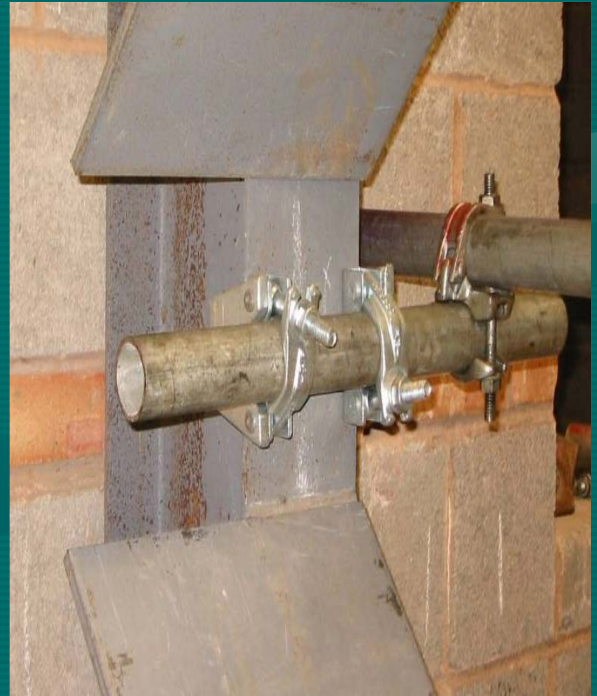
Tie to Steel-work
