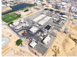
Ajman Sewage Treatment Plant, UAE
