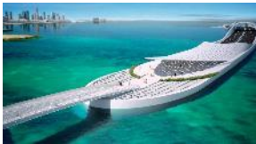
Sharq Crossing, Qatar
