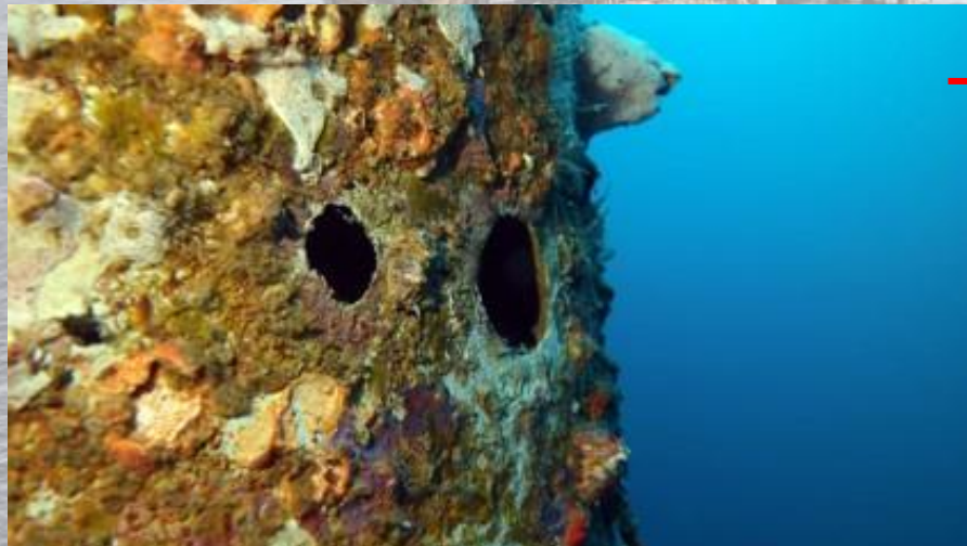
Sea water lift pump caisson picture
