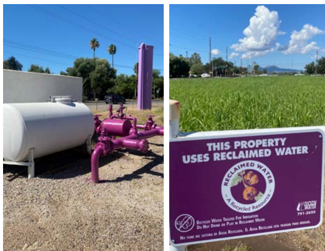
Figure 45. Purple pipes indicating recycled water at the Controlled Environment Agriculture Center, University of Arizona.
