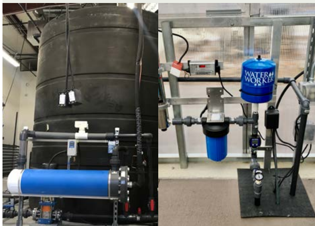
Figure 36. Water tank with UV light disinfection loop (left) and UV loop on underground rainwater tank.
