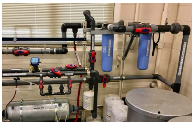
Figure 20. Sediment cartridge filters in blue colored casings, upper right.
