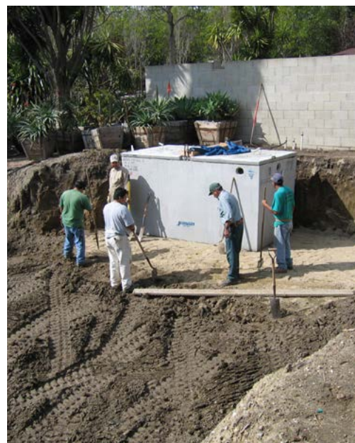
Figure 31. Slow sand filter schematic and during construction.
