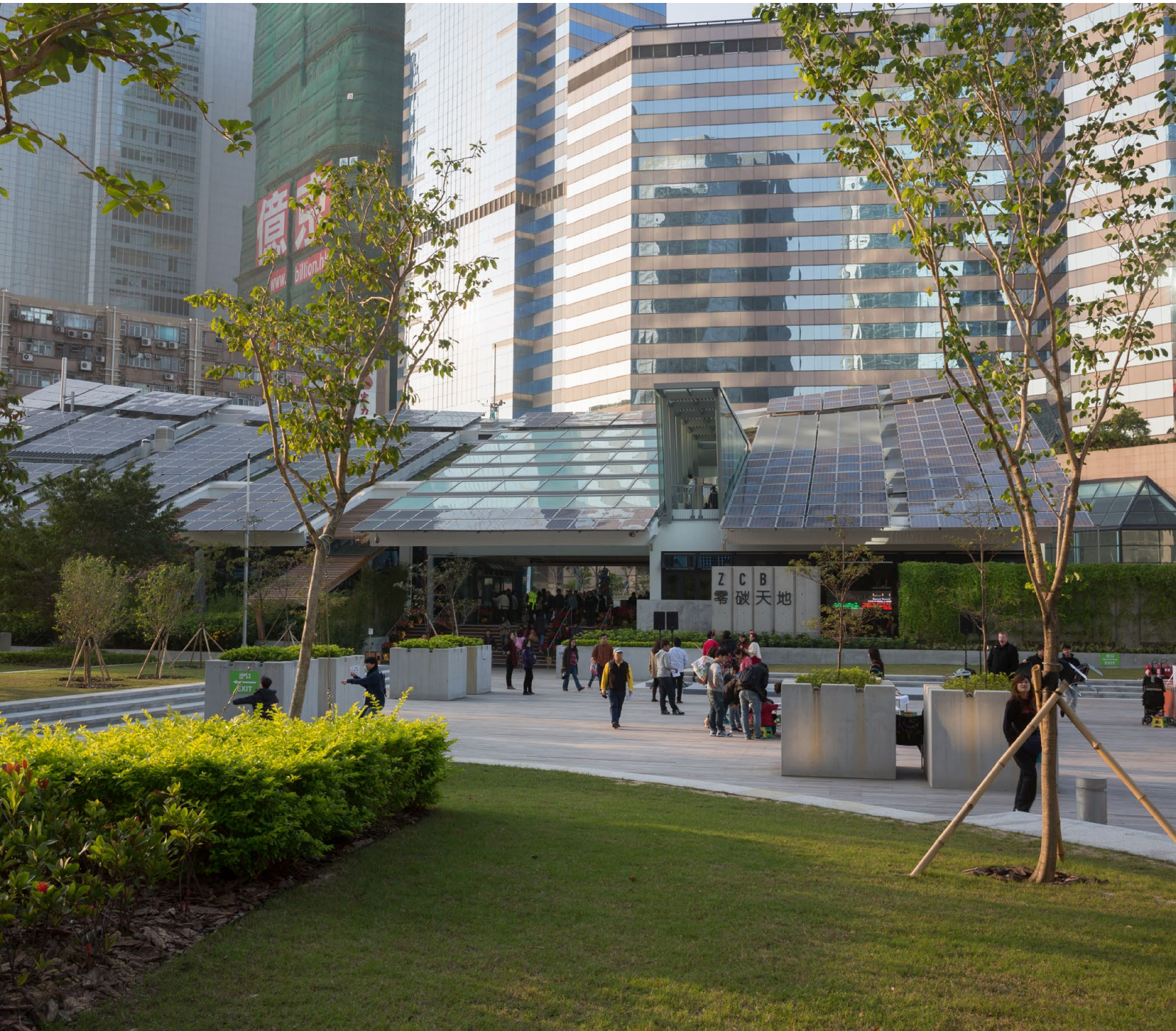
Zero Carbon Building in Hong Kong
