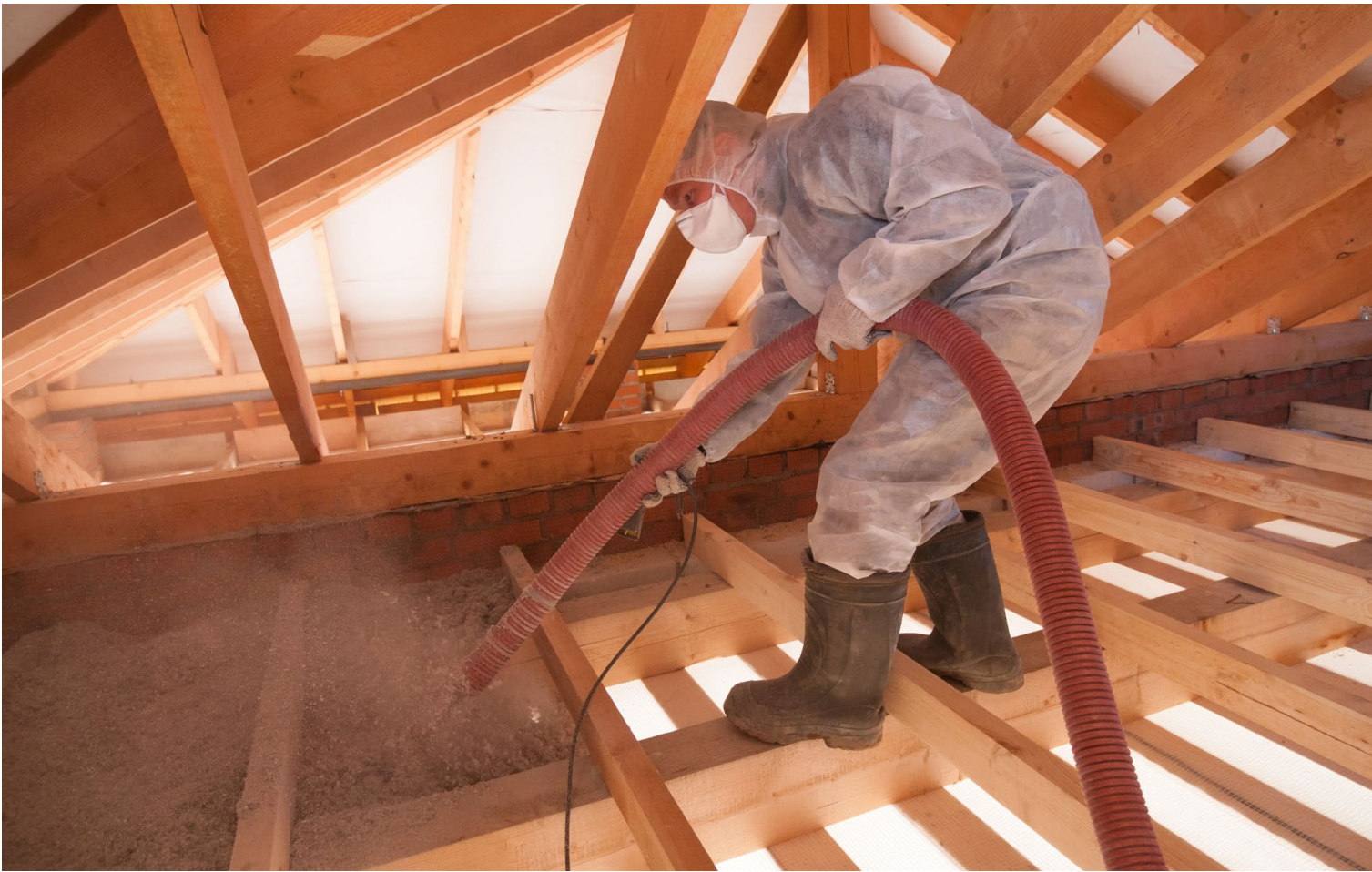
Spraying Eco wool insulation in a home. Policies to incentivize energy efficiency improvements need to overcome underinvestment due to split incentives.
