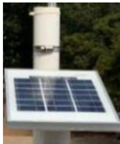
4w/12VDC Solar Panel to connect RTU
