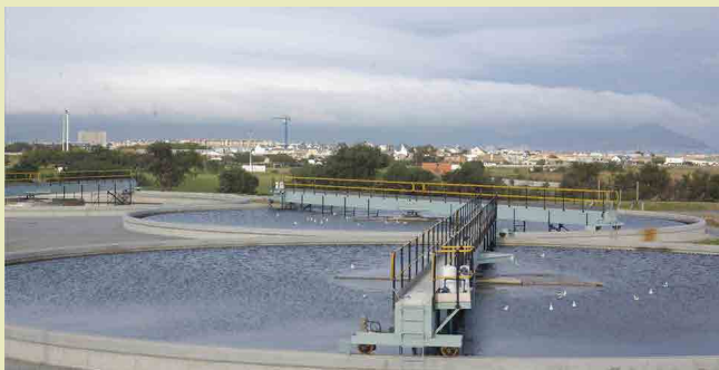
Figure 8: Potsdam wastewater treatment plant, Cape Town
