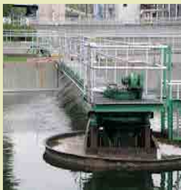
Figure 10: Secondary clarifiers at Polokwane Municipal WWTW
