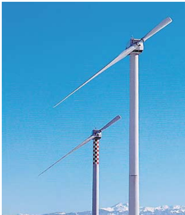
Figure 1.14 - Single-blade with counterweight turbine
