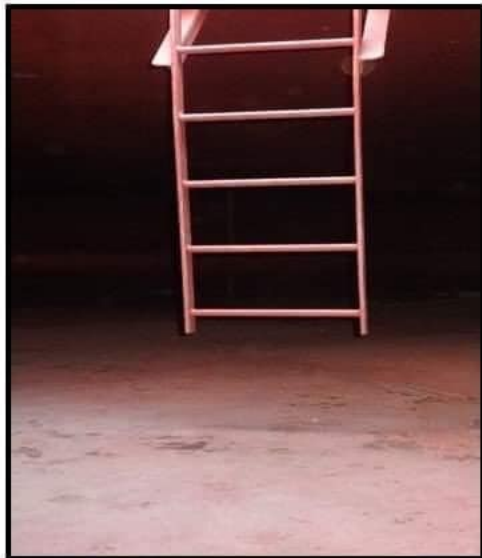
Roof to Tank Ladder
