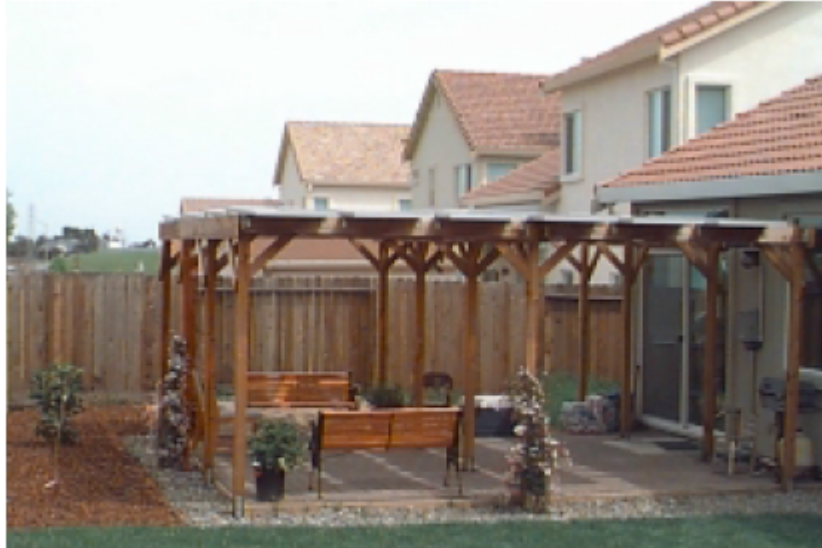
PV mounted on Patio Cover
