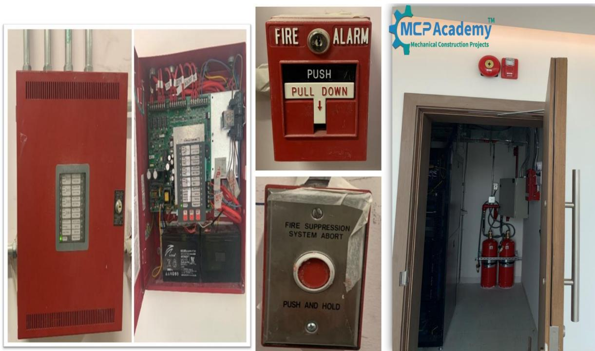
Ensure that the electrical installations and connections such as the locations of the electrical panels and the installation heights for both the Abort Switch and the Manual Release, and that there should be no obstacles to their use
