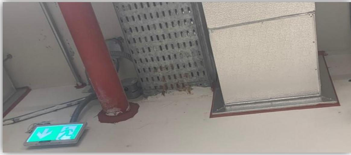
Close all outlets in the walls around the pipes, air conditioning installations and other services that pass inside the room using fire-resistant materials.
