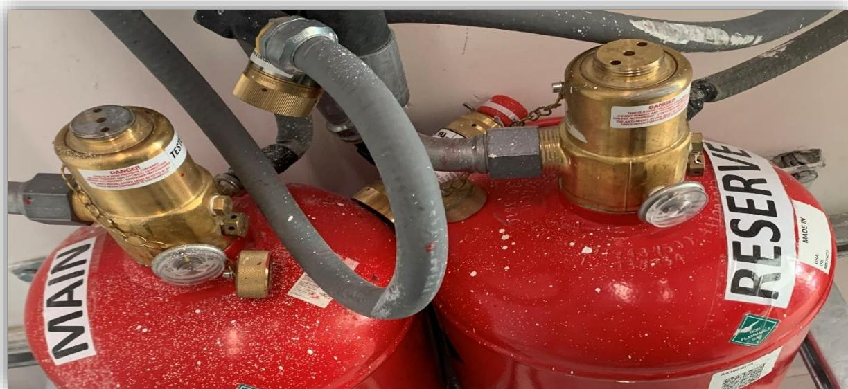
The cylinder head is located on each cylinder, which enables you to install the manual, electric or pressure actuator and is equipped with a cover to protect the cylinder during transportation and installation operations.
