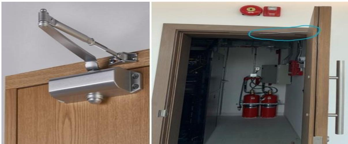
The walls and doors shall be of the approved fire-resistant type and room door holder is required to insure closing case in fire.
