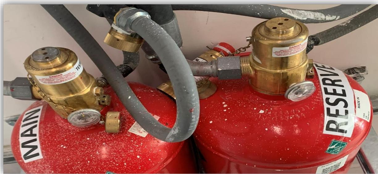
The cylinder head is located on each cylinder, which enables you to install the manual, electric or pressure actuator and is equipped with a cover to protect the cylinder during transportation and installation operations.
