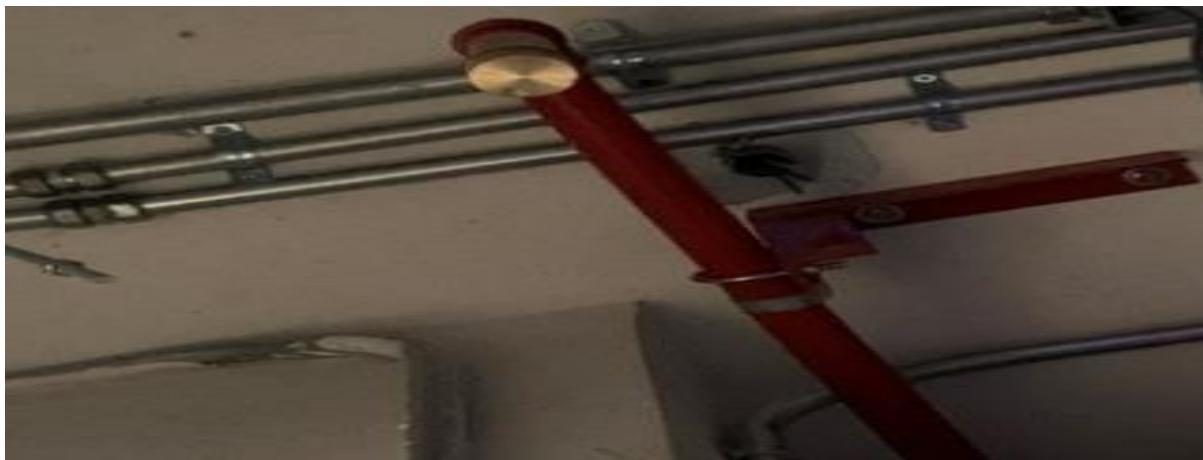
Ensure that the sprinklers are distributed in the room in accordance with the approved plan drawing and that there is no obstruction to their operation
