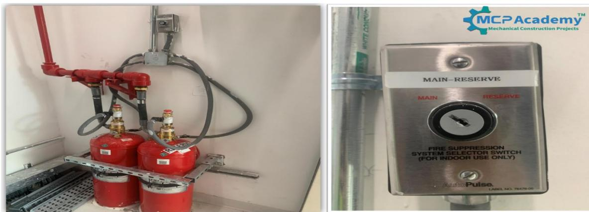
The tests are repeated again on the Reserve cylinders in the system, which are activated by a special key as shown in the picture. The aim of the cylinders is to be a stand by for the main cylinders in the event of maintenance or to recharge the cylinders in their working condition
