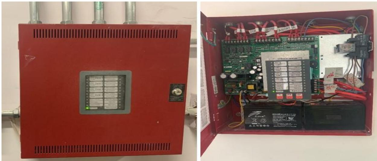
The components of the system such as detectors, bells, sirens and flashers are connected to it and it's work to allow the gas to release by giving a signal to the solenoid actuator start switch when a fire occurs
