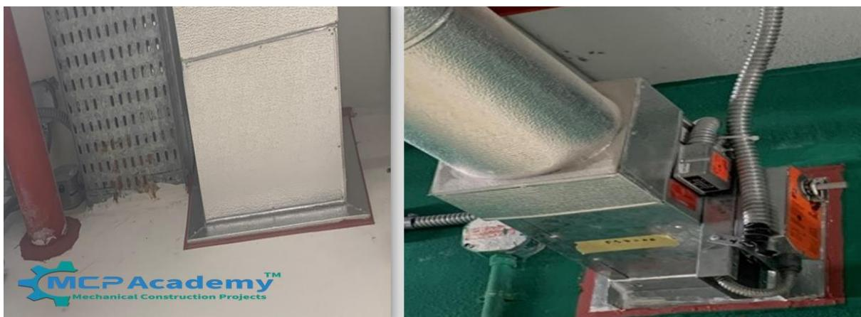
Ensure that all openings between the duct lines, pipes or electrical cable trunk that penetrate the walls of the room are closed using suitable materials to resist fire. Fire Stop Sealant
