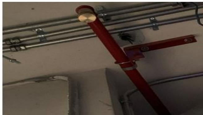
**Discharge Nozzles** work on distributing the gas out of it in the room to be protected. They are made of rust-resistant materials and can withstand high temperatures to resist fire.
