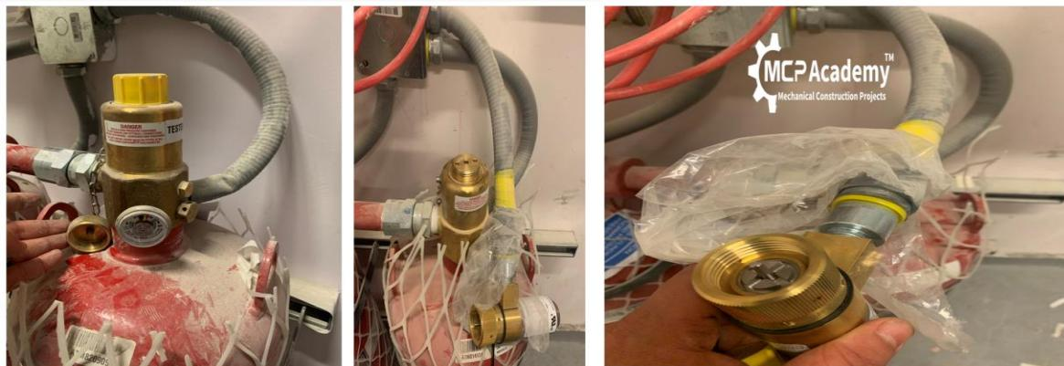
Ensure correct installation of cylinders and cylinder head connections such as supervisor pressure switch and review the data written on the Name Plate of the cylinders
