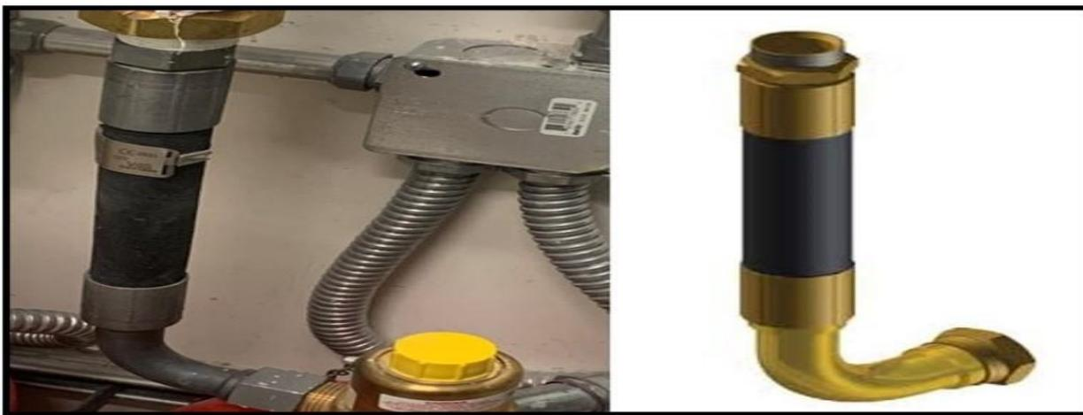
If there is more than one cylinder in the system, the cylinder shall be equipped with a rubber gas discharge hose.
