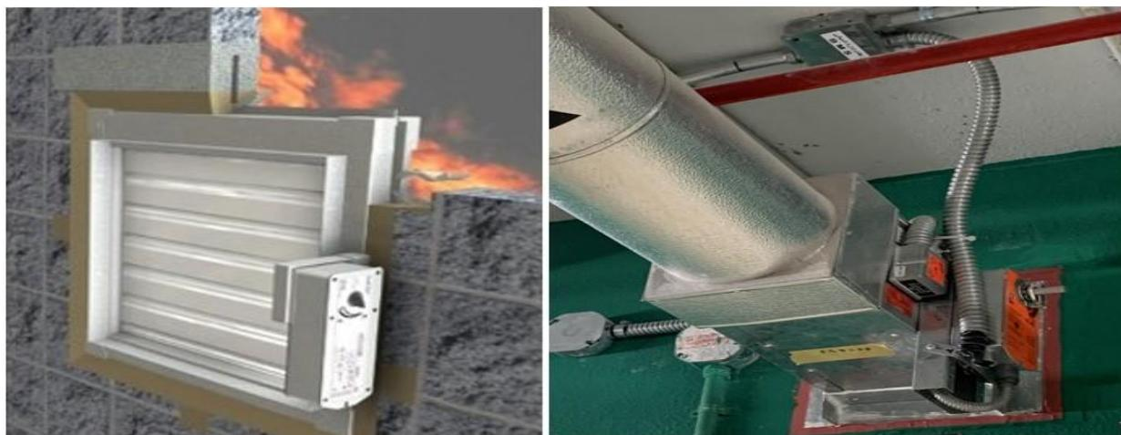
Installing Motorize Fire Smoke Damper HVAC air Duct in the room so that the system can close all of them to prevent gas leakage from the room after gas release
