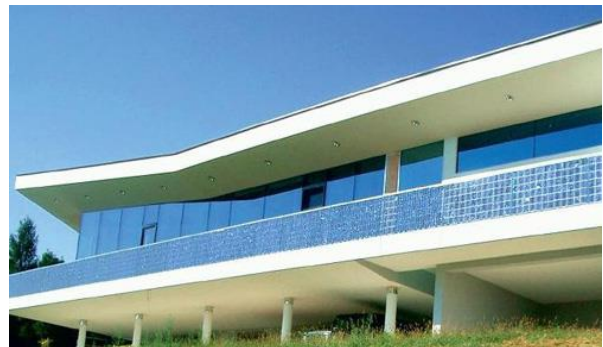
Figure 15 – Externally integrated PV
