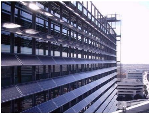
Figure 14 – Externally integrated PV
