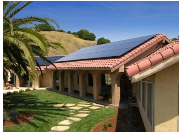
Figure 11 – PV on inclined rooftop (BAPV)
