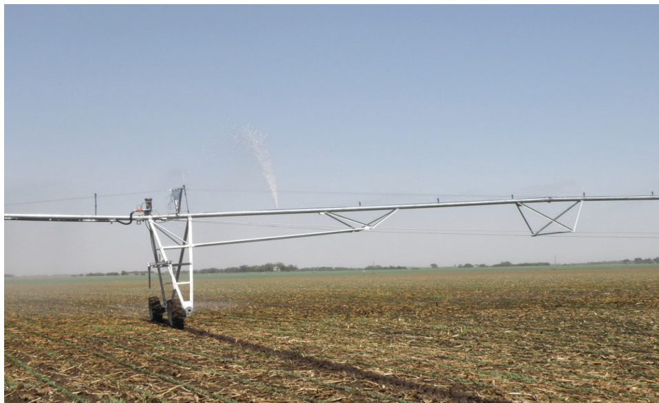
Figure 118. Center pivot with a missing sprinkler.
