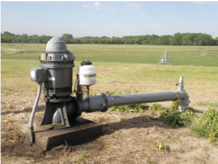
Figure 79. Electric motor for pumping irrigation water.
