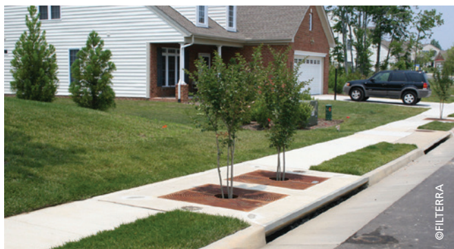
Linear stormwater tree pit
