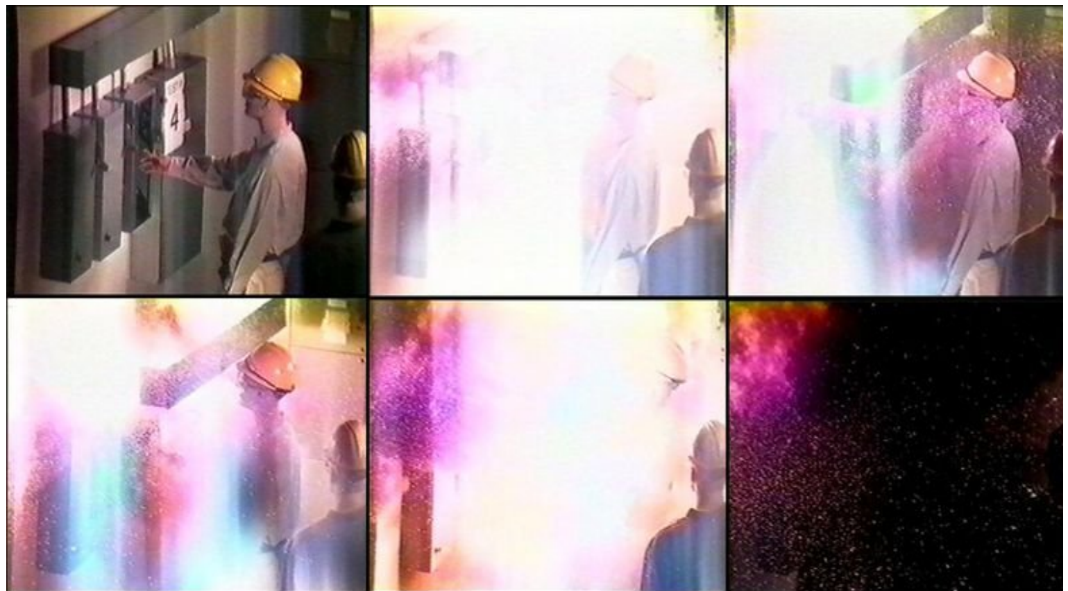
Arc fault explosion on a 480V switchboard with 23kA upstream fault capacity
