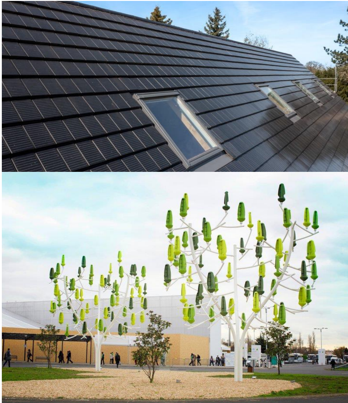
FIG 4 - Solar tiles installed in Germany and a “Wind Tree” by New Wind in France
