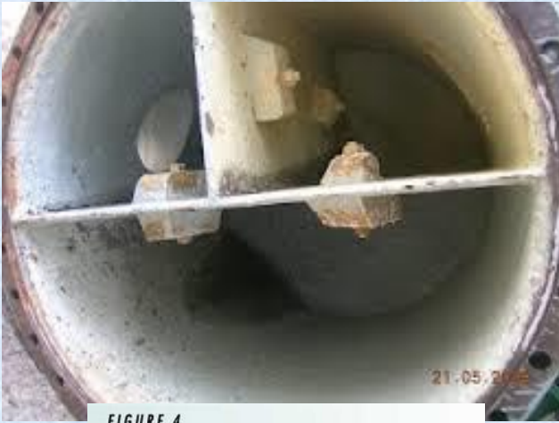
FIGURE 4 WATER BOX CATHODIC PROTECTION
