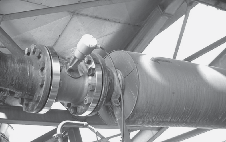
Use the remote version in case of low accessibility to the sensor
