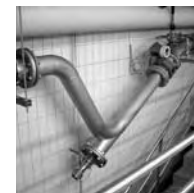
EMF mounted in a siphon
