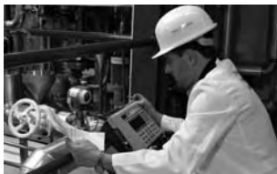
On-site calibration of pressure devices
