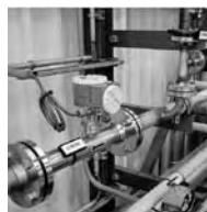
t-mass measuring N 2 consumption
