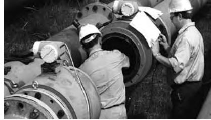
Inspection of the flowmeter pipe
