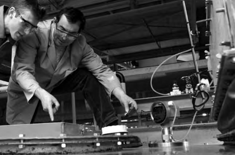
Check of a Levelflex at a chemical plant
