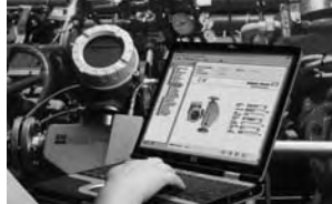
Commissioning and configuration with FieldCare
