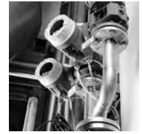
Flowmeters mounted in a fluid riser vertical pipe
