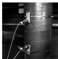
Installation of coated pipes
