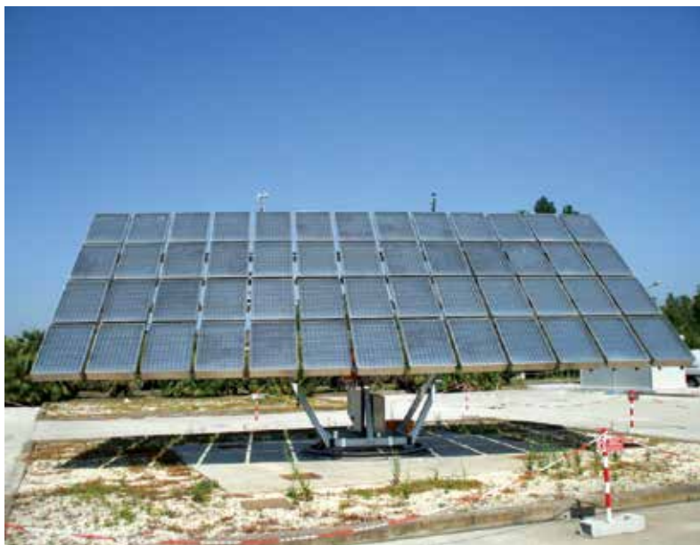
Fig. 14. CPV tracking system in Sun; installation of Rondine™ CPV modules on standard sun-tracker for flat plate modules in Sicily (South Italy). (Courtesy of CPower Srl – www.cpower.it )
