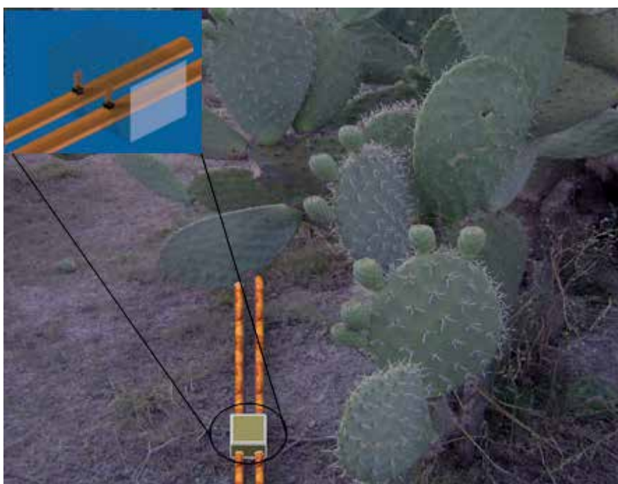
Fig. 16. Conductor in the soil and box connection
