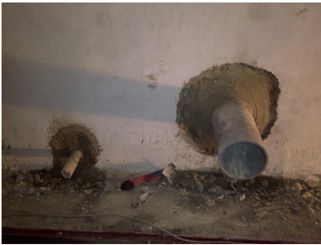
fig-23. Fig-17 pipes through tank walls
