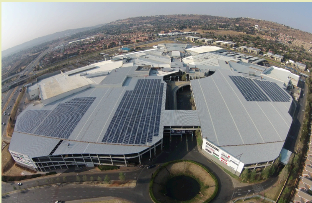
Figure 22: Clearwater Mall 1.5MW of rooftop PV panels – phases 1 and 2
