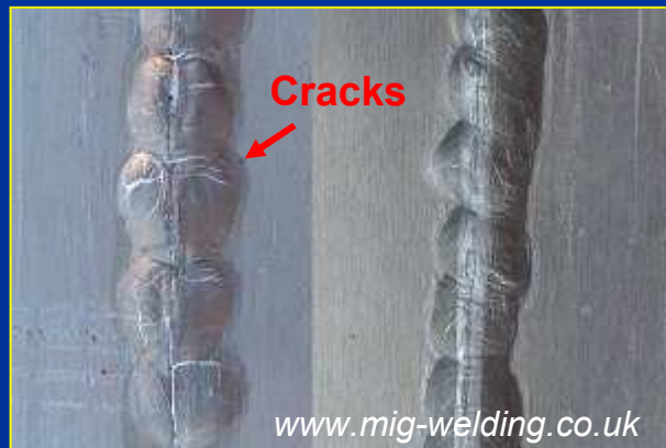
Cracks in aluminium welds
