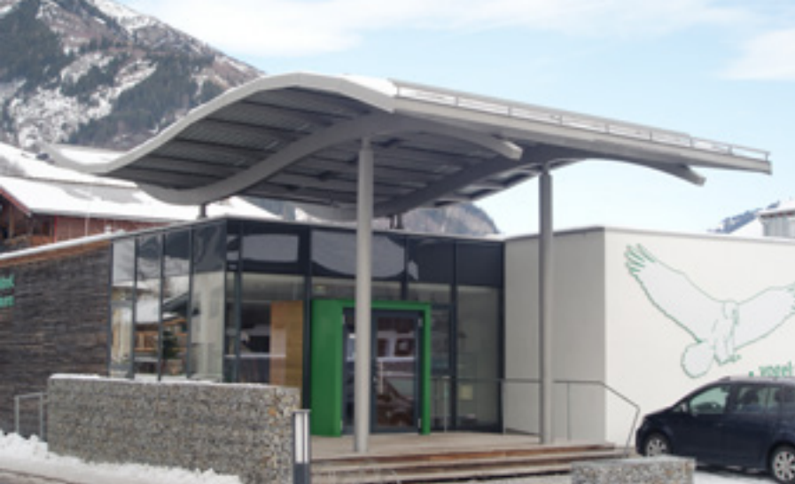
Figure 66: PV wave roof, Rauris
