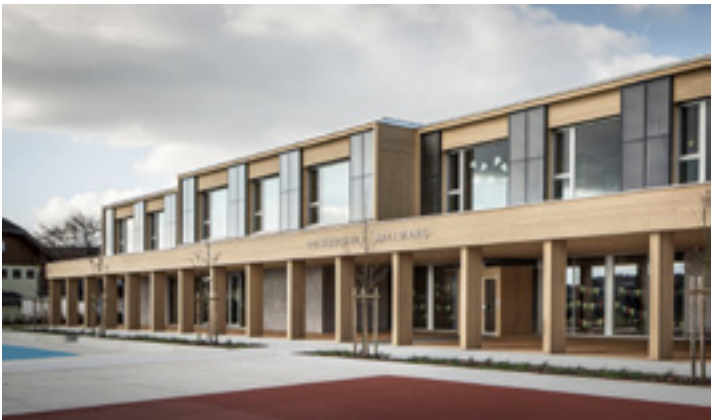
Building-integrated solar thermal system
