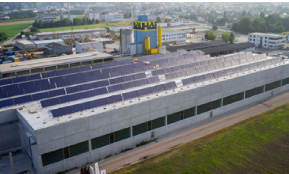
Figure 78: HABAU Concrete Works
