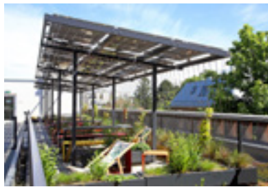
Shading element Combined greening & PV
