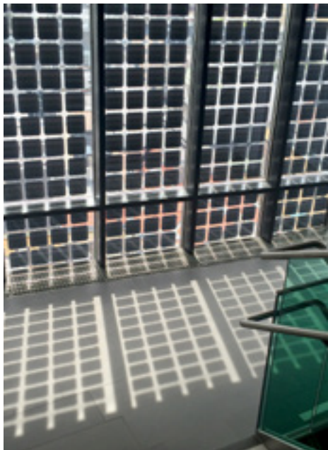
Building-integrated PV Transparent PV Facade-integrated PV
