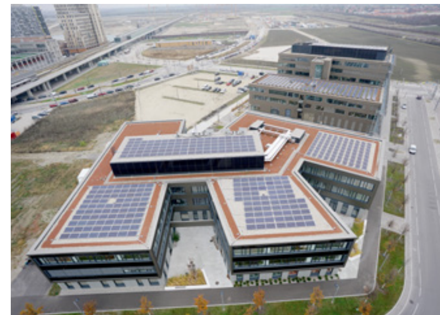
Figure 13: PV system on the roof of Technology Centre 2, Seestadt Aspern
