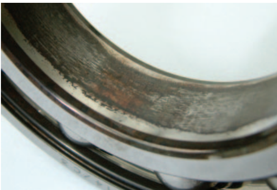
Fretting corrosion on the inner ring
