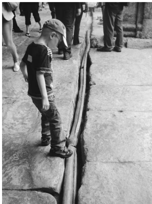
Figure 8.1 Lead pipes were commonly used water distribution lines in antiquity, as in the Roman Aquae Sulis, situated in modern Bath, Britain.
