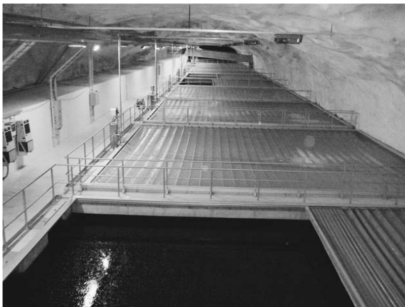
Figure 16.4 Viikinmäki Waste Water Treatment Plant is built underground. The figure shows biological post-filtration. Source: Photograph Rajala, 2007.
