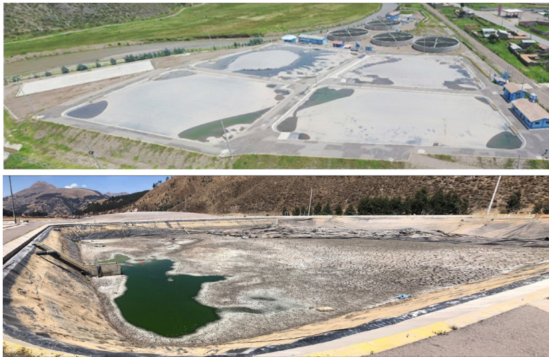
Figure 2.10 Top photo: An anaerobic pond/trickling filter wastewater treatment plant designed for an urban population of 60,000 in Sicuani, Peru. The four geomembrane-covered anaerobic ponds are operated in parallel, with the generated biogas burned in a flare rather than used as an alternative energy source. The anaerobic ponds were chosen to save area since the available land for wastewater treatment was limited – a common problem in small cities where wastewater treatment is not taken seriously by local governments. Bottom photo: After 5 years of operation, the geomembrane on one pond was removed for desludging. At the time of this writing, the pond had been uncovered and out of service for more than 6 months as plant personnel searched for an affordable solution for desludging and final disposal, neither of which were included in the original design or operations manual. Source: Photos courtesy of CONASIN SRL, Cusco, Peru.
