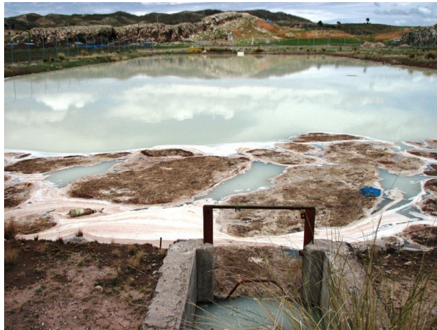
Figure 3.2 A facultative pond receiving domestic wastewater from the municipality of Huata, Peru (Population ~1600) overloaded by discharges of cheese processing wastewaters. In this case, a small cheese processing plant had much stronger wastewater than the design population.
