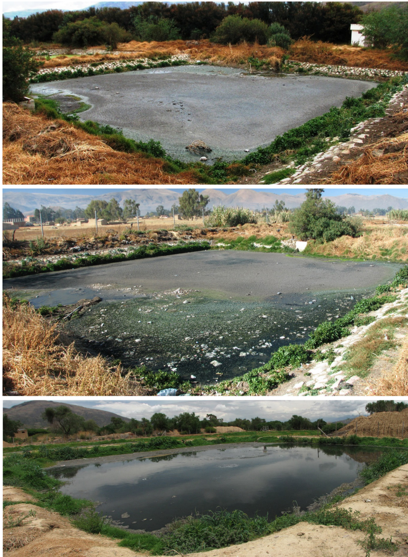
Figure 2.11 Common examples of abandoned anaerobic ponds without methane capture, without a desludging plan, and without maintenance (top to bottom: Arani, Punata, and Tarata, Bolivia).
