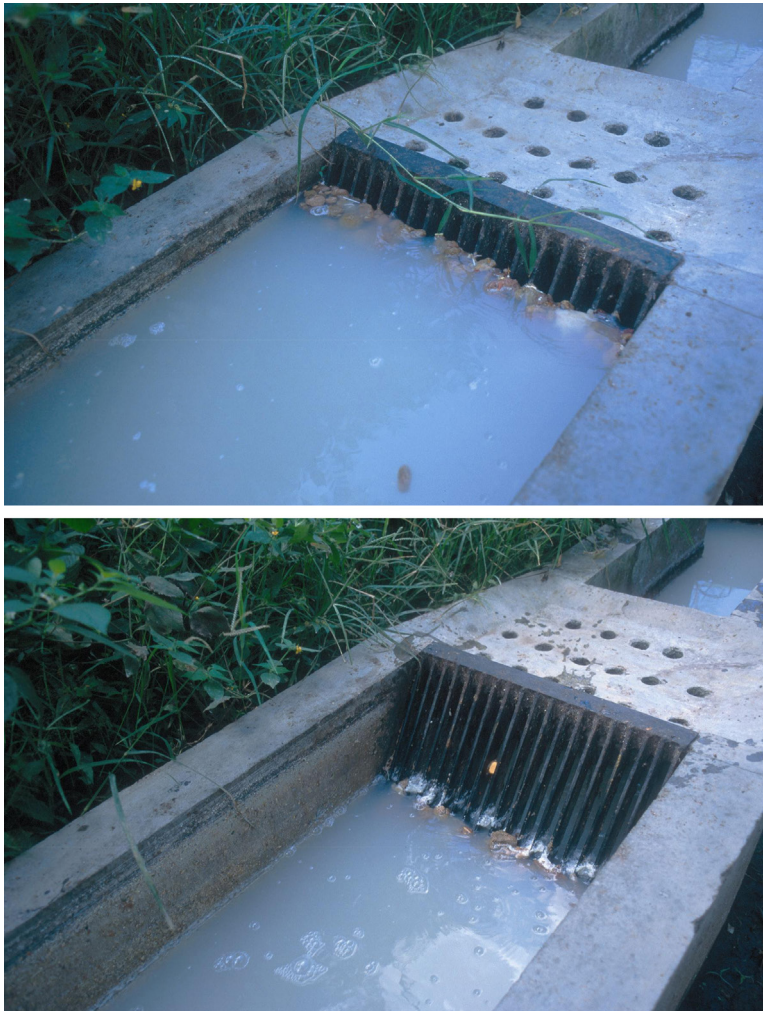
Figure 4.5 The timely removal of screenings is a fundamental operational task to maintain uninterrupted flow through the grit chamber. A bar screen has to be cleaned daily or even hourly depending on the raw wastewater characteristics. The top photo shows the water level 24 hours after cleaning the bar screen, while the lower photo shows the level right after cleaning the bars. This bar screen should have a bypass channel (Figure 4.6). The retained solids are human feces that should pass through the bars to be treated in the wastewater treatment plant (Urbanización Alpes Suiza, San Salvador, El Salvador).
