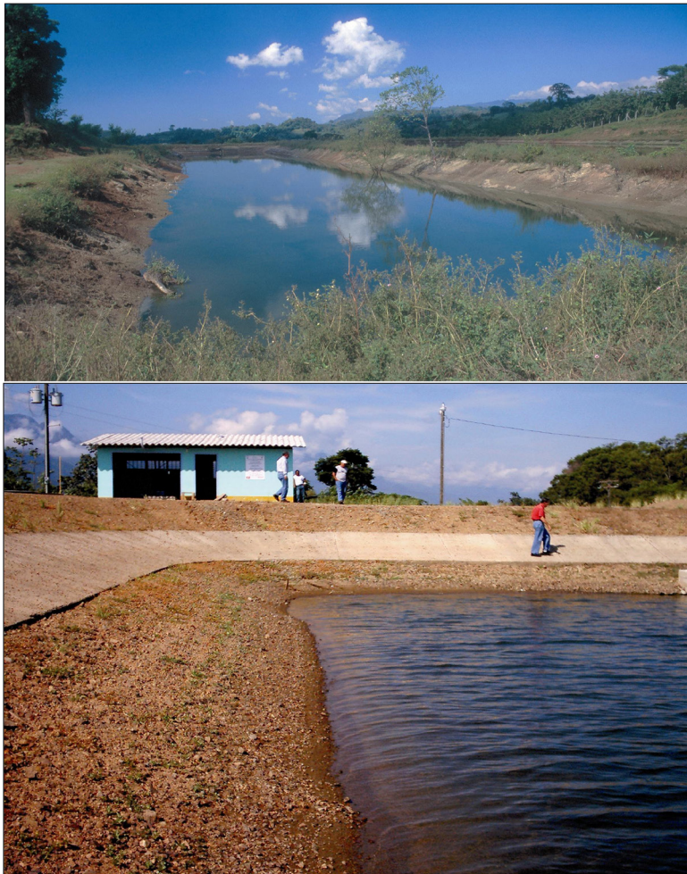
Figure 9.4 Examples of the importance of the water balance and the effects of poor construction. In both ponds, the infiltration losses are excessive and water levels cannot be maintained. Both ponds lack impermeabilization on the bottom and interior embankment slopes (top: Zaragoza, El Salvador; bottom: La Ceiba, Honduras. Bottom photo courtesy of Ing. Iván Olivieri).
