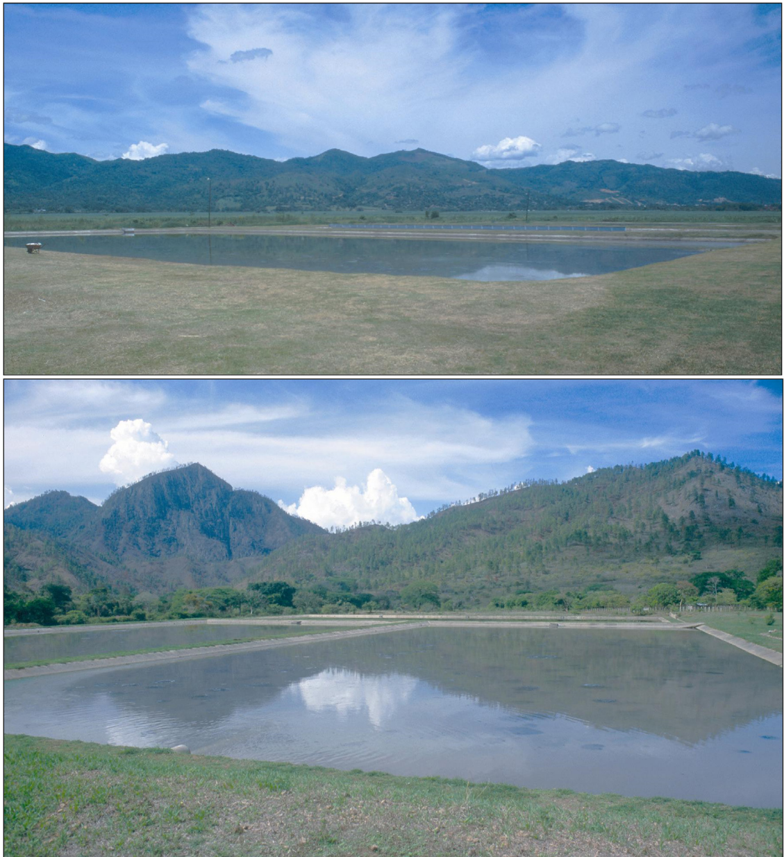
Figure 9.1 Examples of well-constructed and maintained pond systems. The embankments are well maintained with the grass routinely cut. The interior slopes have a concrete revetment that serves to control growth of aquatic plants at the shoreline and prevent erosion by wave action. The surface of the water has no floating materials or scum, and the water level is maintained in the center of the revetment (top: Villanueva, Honduras; bottom: Danlí, Honduras).
