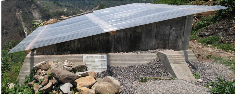
Figure 8.8 The existing reservoir at the San Antonio, Sololá wastewater reuse project has an estimated maximum volume of 50 m 3 and was designed for a pilot irrigation project of 1.84 ha.
