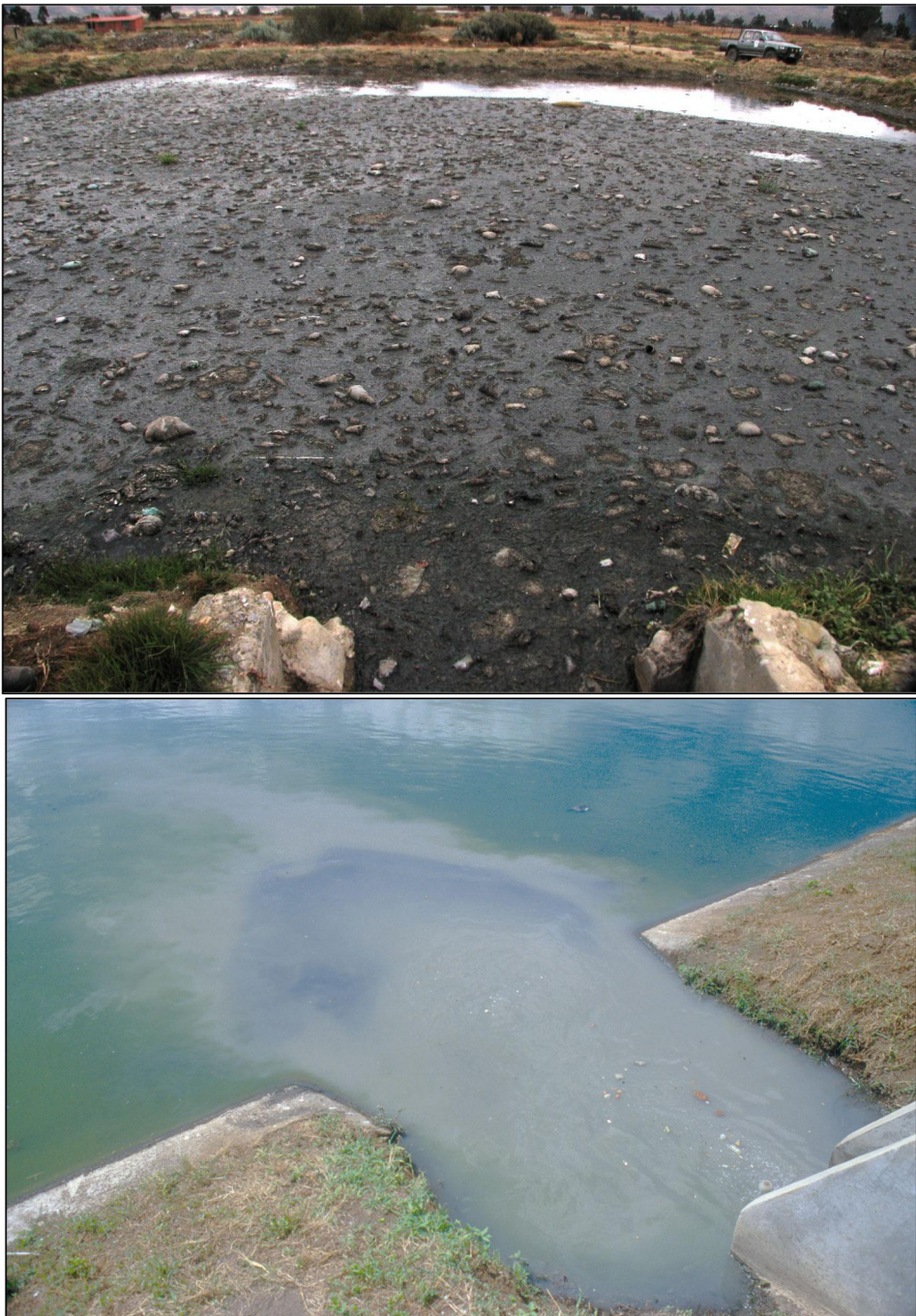
Figure 2.2 Examples of screenings and grit accumulation in primary waste stabilization ponds designed and built without considering preliminary treatment. Screenings and grit contain high concentrations of excreted pathogens and must be disposed in a sanitary manner onsite or offsite. Top: Punata, Bolivia. Bottom: Chinendega, Nicaragua.
