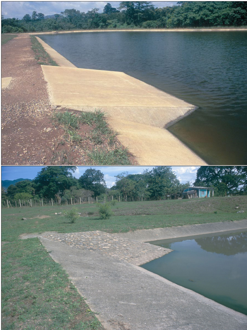
Figure 9.29 Examples of access ramps for sludge removal in primary ponds. Top photo: facultative pond, Santa Cruz de Yojoa, Honduras. Bottom photo: anaerobic pond, Danlí, Honduras.
