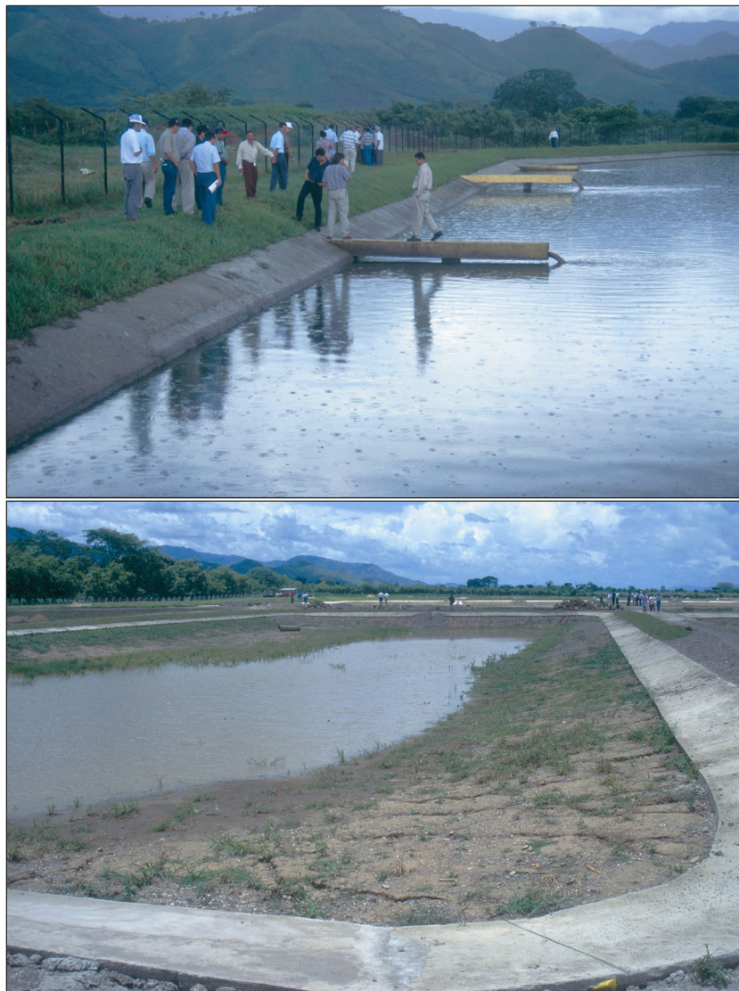
Figure 9.27 Examples of well-built pond revetments. The photo above (Catacamas, Honduras) shows the new revetment built for the pond shown in Figure 9.26 after rehabilitation. The photo below shows a well-built revetment for a maturation pond (Catacamas, Honduras).
