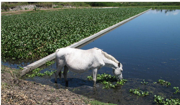
Figure 10.9 Water hyacinths covering 50% of a maturation pond, with the baffle preventing further spread. The hyacinths were placed intentionally with the mistaken belief that they would improve treatment. Hyacinths are prime habitat for insects and should be removed immediately if they begin to grow in ponds. Domestic animals should not be permitted inside the treatment plant installation.
