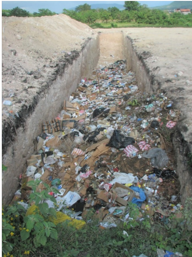
Figure 4.18 Municipal solid waste is deposited in this trench at Villanueva, Honduras. When full, the trench is backfilled and excess soil is used for other purposes onsite. The same procedure can be used at larger wastewater treatment facilities for preliminary treatment solids and should be included in the original design of the system.
