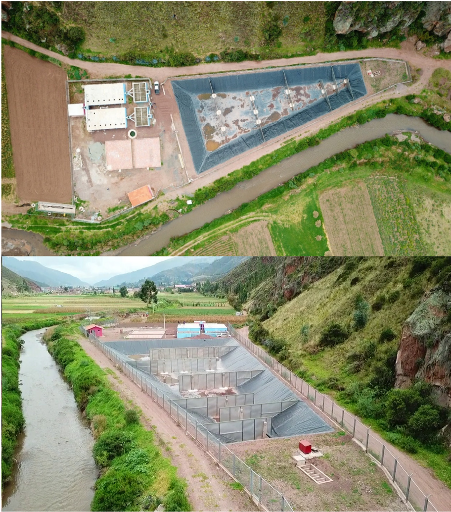
Figure 6.1 A maturation pond following an anerobic reactor with river discharge. A pond system with agricultural reuse was originally proposed for this municipality, but the mayor chose this small area, the worst possible site, as the only available for a wastewater treatment plant. Groundwater is at river level, and a pump station had to be installed to pump to the elevated anaerobic reactors. The maturation pond design water depth is 1.5 m, with a hydraulic retention time of 2.8 d. After three years, the system is still not in operation (2021), and most likely will be abandoned. The plant was built to satisfy the requirement of wastewater treatment. Photo courtesy of CONASIN, SRL, Cusco, Peru.
