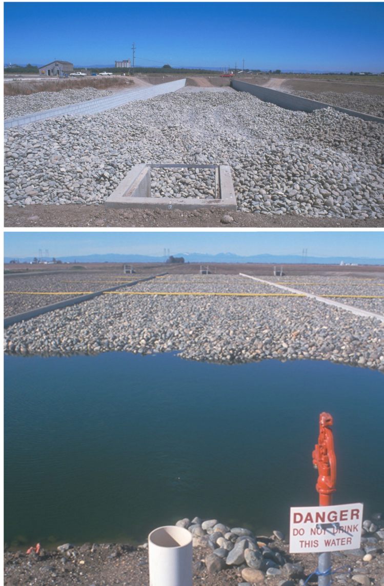
Figure 6.6 A rock filter installation in the city of Biggs, California. Top photo: filter construction with river rock, ranging in size from 8 to 15 cm, with void a volume equal to 40% of total volume. Bottom photo: Three parallel batteries of filters in operation. Rocks must be above water level to avoid algal growth on the surface.
