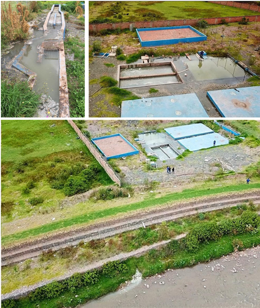
Figure 3.7 This wastewater treatment plant was designed and built without flow monitoring using population and per capita estimates for the design flowrate. Within a year after construction, the plant, which never had an operator, was inundated: first, the grit chamber filled and overflowed; next, the wastewater flowed over the anaerobic reactors and filled and clogged the media filters; after overflowing the filters, it drained into a sump with a gravity discharge pipe to the river – a case of wastewater flowing over the treatment facility rather than through it. Photos courtesy of CONASIN SRL, Cusco, Peru.
