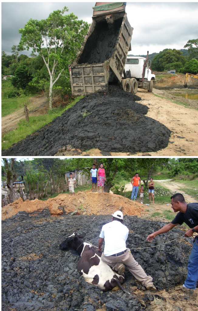
Figure 7.5 Sludge from a drained facultative pond being disposed on the pond's embankment. This pond in Tela, Honduras, had operated for 15 years, and no plans had ever been made for sludge removal, drying, and storage. When the pond finally needed desludging, the only space available for disposal was the embankment. As a result, the neighboring population, which had open access to the pond installation along with domestic animals, was put at high risk. Viable helminth eggs in the pond sludge after draining ranged from 0.4 to 25 eggs/g dry weight, and one sample taken on the embankment measured 5.1 eggs/g (Oakley et al. , 2012). The prevalence of soil-transmitted helminth infections in Honduras ranges from 20 to 50% (Figure 7.3).
