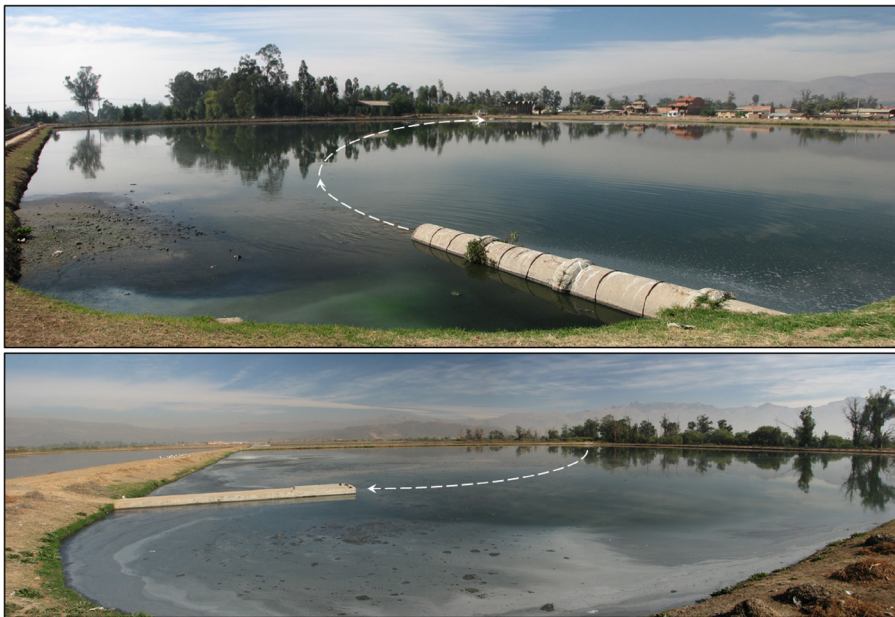
Figure 5.28 The inlet (top) and outlet (bottom) of facultative pond LP1 (Figure 5.24). The single inlet/outlet locations in a rectangular pond caused significant hydraulic short circuiting with large dead spaces in much of the volume, and sludge accumulation along the shoreline to the left of both the inlet and outlet in the direction of flow. Note the sludge accumulation to the left of the inlet (Albarrancho Wastewater Treatment Plant, Cochabamba, Bolivia).
