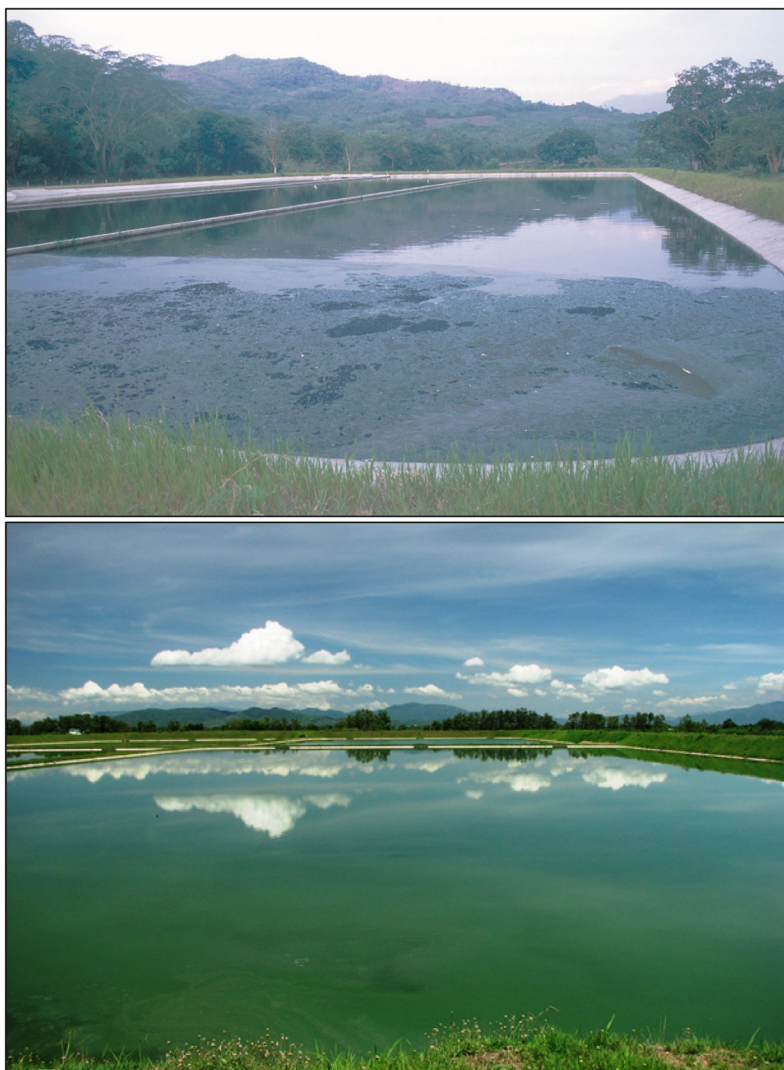
Figure 5.16 Top photo: The facultative pond at Trinidad, Honduras, was anaerobic throughout the monitoring project as a result of a short hydraulic retention time, sludge accumulation, and use of baffles that caused the inlet to be organically overloaded. Bottom photo: The facultative pond at El Progreso, Honduras, is an example of a well-designed and operated facultative pond, with brilliant green color from the algal growth. The pond is free of odors and has no floating scum or aquatic plant growth. Both ponds had similar BOD 5 removal.
