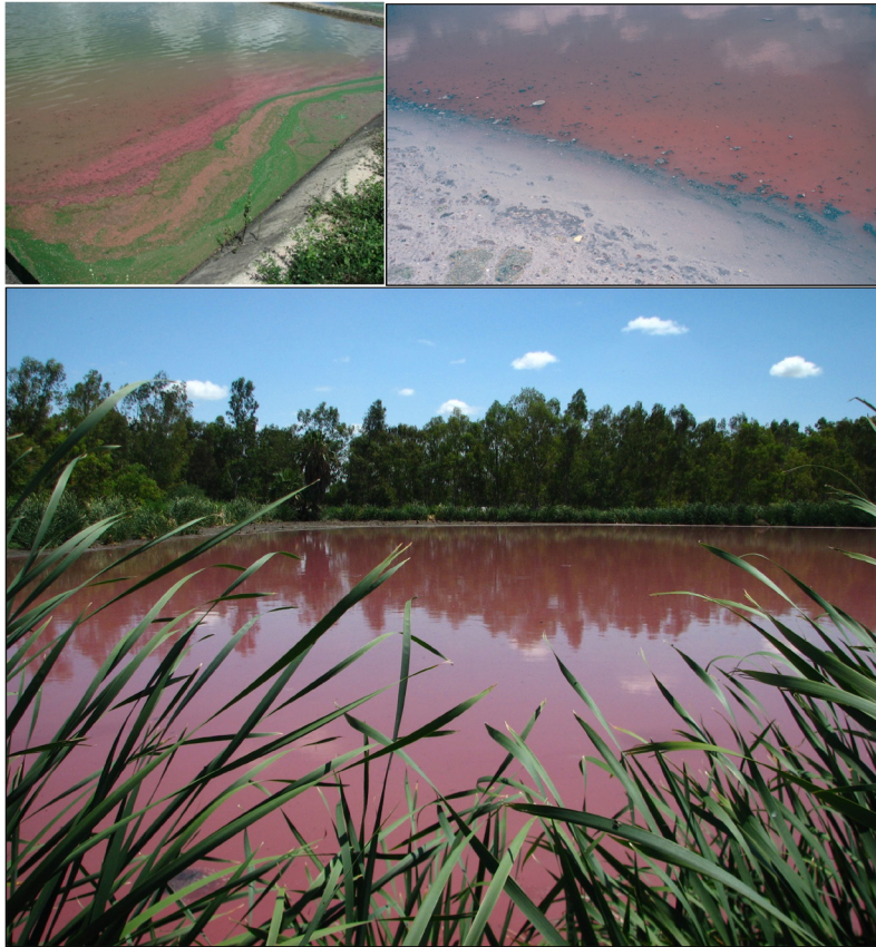
Figure 5.8 Examples of reddish coloration in facultative ponds as a result of anoxygenic photosynthesis by the purple and green sulfur bacteria. The top left photo is the dead space in a corner of an otherwise well-functioning pond. The top right photo is a highly overloaded pond converting to an anaerobic one. Bottom photo is an overloaded pond (top left: Lagarto, Brazil; top right: Villanueva, Honduras; bottom: Mendoza, Argentina).
