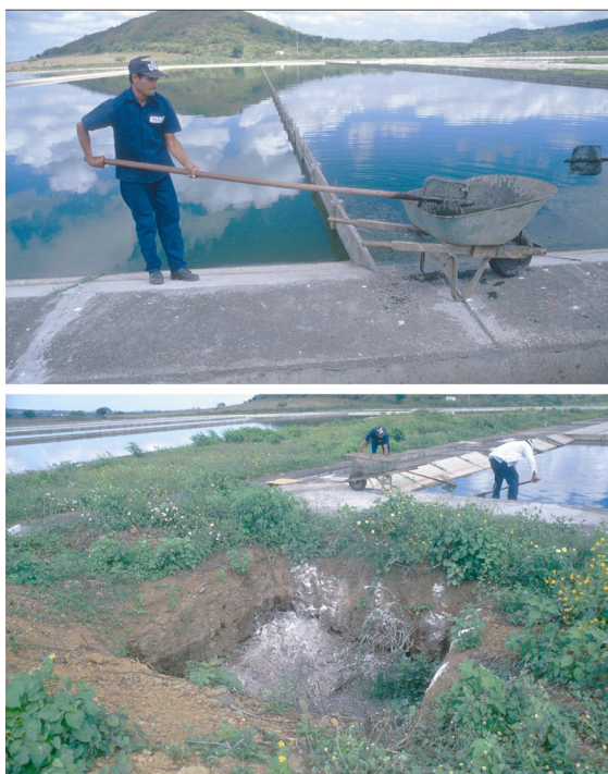
Figure 10.5 Floating scum and solids accumulate in corners, where the operator can easily remove them with a scum rake and put them in a wheelbarrow. Afterwards, they must be buried, or covered with a layer of soil or lime. In the photo below the operators put the collected scum solids in a small excavation and cover them with lime to control odors. When the excavation is filled, it is covered with a layer of soil (Masaya, Nicaragua).
