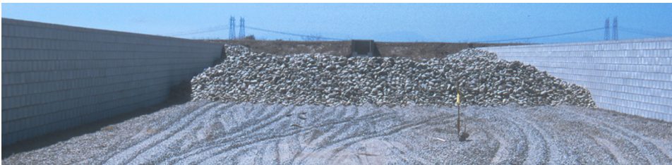
Figure 6.17 Rock Filter 1 under construction. The three filters in parallel were designed for a water depth of 2.0 m, with 0.2 m of filter above the water surface, with a design \text{HLR}_{\text{filter}} = 0.15 \text{ m}^3/\text{m}^3 \text{ d} . See also Figure 6.6.
