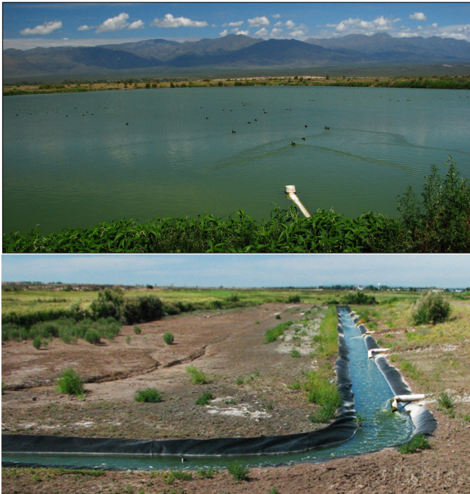
Figure 7.29 Top photo: One of the 12 secondary maturation ponds in parallel at the Campo Espejo waste stabilization pond system. Based on the design in the mid-1990s to meet the 1989 WHO guidelines for agricultural reuse, each primary and secondary maturation pond has a hydraulic retention time of 6.15 days at the design flowrate of 129 600 m 3 /d or 10 800 m 3 /d per pond. Bottom photo: One of the several final effluent discharge canals that feed the network of smaller irrigation canals for the entire 3000 ha Campo Espejo ACRE, all by gravity flow. The effluent also meets the 2006 WHO guidelines for restricted irrigation: For crops eaten cooked that have contact with wastewater, a 30-day waiting period after cessation of irrigation is required before harvest to allow pathogen die-off from natural mortality; for crops eaten uncooked, the contact with treated wastewater is strictly prohibited (e.g., fruit trees).
