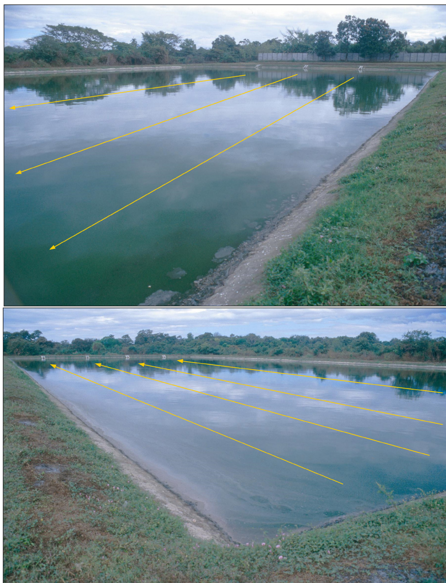
Figure 9.14 Multiple inlets (photo above) and outlets (photo below) are used in facultative ponds to approximate plug flow. Baffles cannot be used in facultative ponds because of the need to disperse the influent throughout the pond area where solar insolation promotes photosynthesis and oxygen production. Multiple inlets also promote the uniform distribution of deposited sludge in the first 30% or so of the pond's length (Chinendega, Nicaragua).
