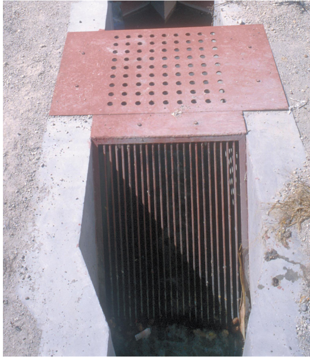
Figure 4.4 A well-designed bar screen should have rectangular bars with widths of 5–15 mm and thicknesses of 25–40 mm, with a drainage platform to drain the retained coarse solids – which have a water content of \geq 80\% – before sanitary disposal. A spacing between the bars of 50 mm is recommended, so that human feces pass through the grate without being retained (see Figure 4.5 ). The inclination with the horizontal should be between 45 and 60°, so that the retained material is easily removed with a rake. The construction material of the bars and the drainage platform should be corrosion-resistant metal such as stainless steel, galvanized steel, or aluminum (Alta Vista Urbanization, San Salvador, El Salvador).
