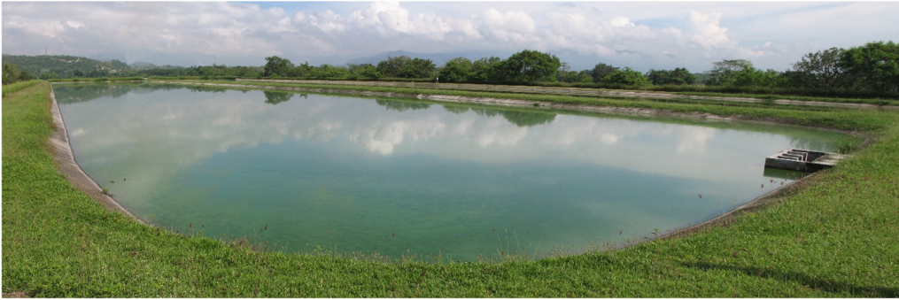
Figure 6.8 An unbauffed maturation pond with l/w = 5.4/1 (285 m \times 53 m), with the inlet at the water surface. Short-circuiting is not apparent, but monitoring data are not available and performance cannot be assessed, a common problem. (Choloma, Honduras).
