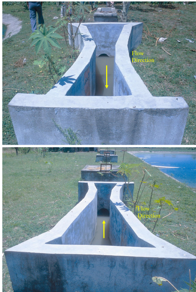
Figure 4.14 Another example of a poorly designed and constructed Parshall flume without free-flow (Choloma, Honduras). Pre-fabricated Parshall flumes are always recommended to avoid this common problem.
