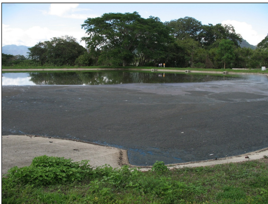
Figure 5.7 A continuation of the process shown in Figure 5.6 . Rising sludge from excessive accumulation is gradually covering a facultative pond. This pond operated for more than 15 years without desludging and is now anaerobic, with the maximum release of methane into the atmosphere (El Paraiso, Honduras).
