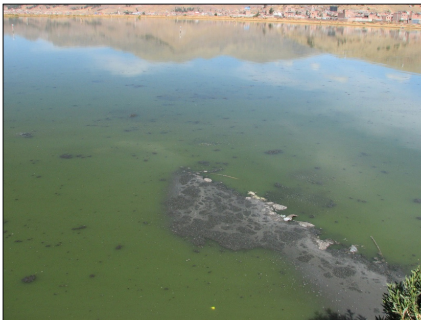
Figure 5.6 Rising sludge from the anaerobic zone lifted with methane and carbon dioxide bubbles. This facultative pond had excessive sludge accumulation after more than 20 years of operation without sludge removal. In spite of the accumulation, the aerobic zone is still functioning well as seen by the bright green color. Unless the pond is desludged, the rising sludge will eventually cover the surface and the pond will turn anaerobic throughout its depth (Figure 5.7; Puno, Peru).
