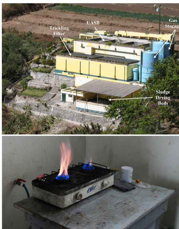
Figure 2.16 A well-designed and built UASB/trickling filter wastewater treatment plant that has operated for over 25 years in Sololá, Guatemala. The produced biogas is used for cooking in various houses near the plant, and a maximum of 24 ha is irrigated with the effluent during the growing season. Unfortunately, a batch stabilization reservoir was never built, and the final effluent has concentrations of E. coli measured at 1.2 \times 10^7 MPN/100 mL, posing serious health risks to the farmers, their families, and local consumers (see Section 7.2.2, pp. 205–211).
