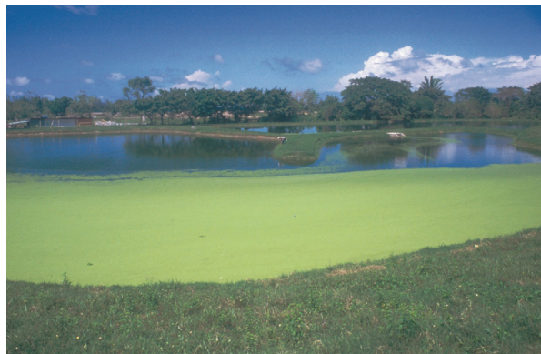
Figure 10.8 A common example of duckweed, carried by the wind or by birds, that has partially covered the surface of a maturation pond. The operator should remove the duckweed as soon as possible before the pond is entirely covered. Domestic ducks rapidly eat duckweed and a few can be brought to a heavily covered pond to aid in its removal (Tela, Honduras).
