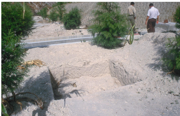
Figure 4.9 An excavation next to the bar screen and the grit chamber to bury the solids collected daily. The design of the pretreatment facility should include a reserved area close-by where the operator can bury screenings and grit solids with minimal handling. Pretreatment solids will always be contaminated with pathogens, and screening solids are unsightly with noxious odors like bad smells and bad looks. Bar screen solids need to be buried daily, while grit solids require burial only when cleaning the grit chamber (Urbanización Alta Vista, San Salvador, El Salvador).
