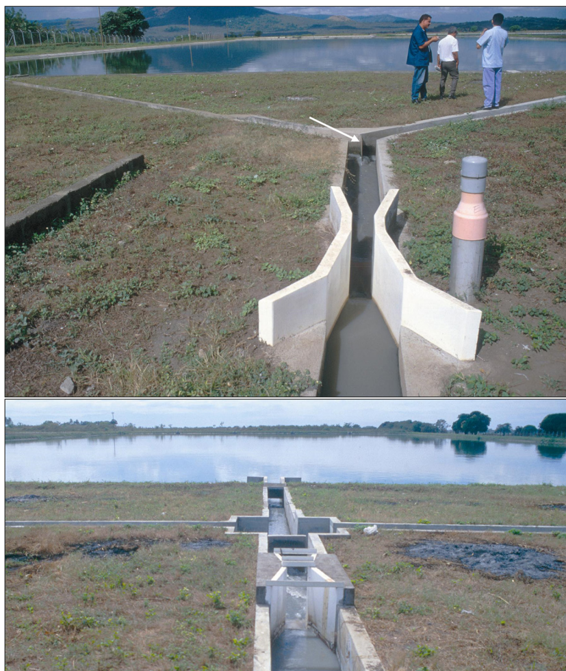
Figure 9.17 Examples of flow devices for adjusting the distribution of flows among multiple entrances in facultative ponds. In the top photo (Masaya, Nicaragua), an adjustable partition (arrow) that can easily be moved by hand is used. In the bottom photo (Chinendega, Nicaragua), a distribution chamber that cannot be adjusted is used; in this case the chamber has to be built and leveled with precision. In both cases, prefabricated Parshall flumes are used to measure the flow distribution accurately between ponds in parallel. Also note the use of open channels to facilitate flow distribution adjustment and channel maintenance.
