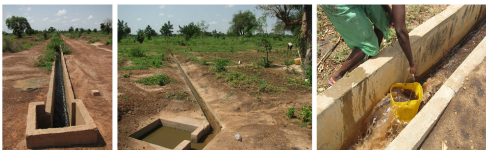
Figure 7.16 Left photo: The main irrigation canal receiving the final effluent. Middle: Smaller canals fed from the main canal conveying effluent to small plots. Right photo: Effluent is taken from the canals in buckets to irrigate crops. (Source: Right photo courtesy of Nitiema et al. 2013).
