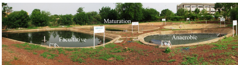
Figure 1.30 The anaerobic–facultative–maturation waste stabilization pond system at the International Institute for Water and Environmental Engineering (2ie), Ouagadougou, Burkina Faso. The system treated domestic wastewater for a population equivalent of 448 persons, with a mean flowrate of 55 m 3 /d, and a theoretical hydraulic retention time of 18 days.
