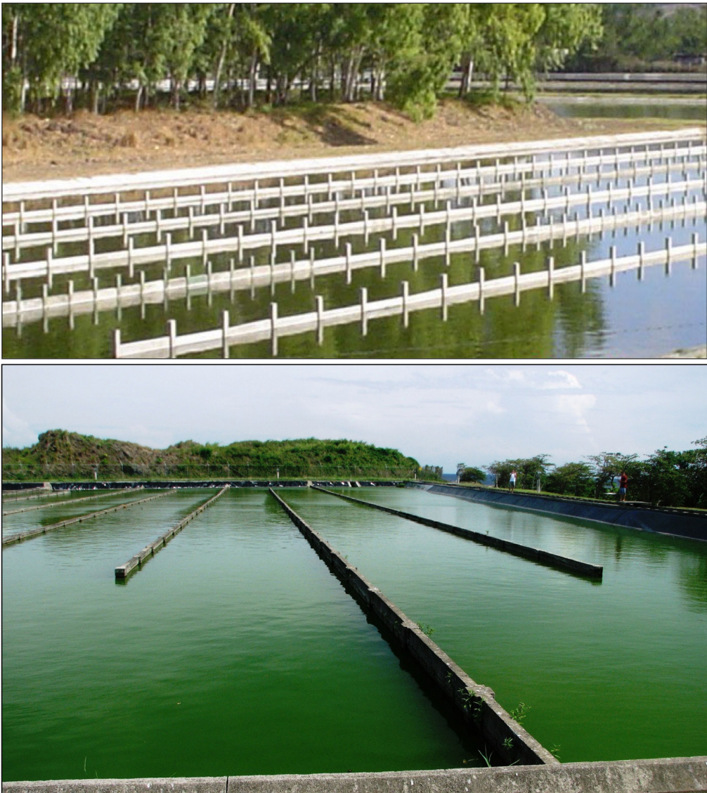
Figure 9.15 Examples of baffled maturation ponds using a single inlet and outlet to promote plug flow. Baffled maturation ponds should have a minimum length/width ratio of 50 to 1. In the top photo (Estelí, Nicaragua), the longitudinal channels have a length/width ratio \approx 100/1 . The bottom photo (Roatán, Honduras) shows transverse baffles, which better minimize the effects of wind at this site (top photo courtesy of Ing. Italo Gandini).
