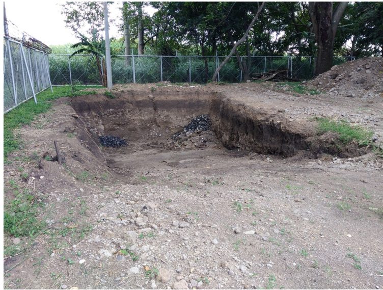
Figure 7.7 An excavation for disposal of dewatered sludge at the Lagos de Lindora wastewater treatment plant, San Jose, Costa Rica. In areas where excreta-related disease prevalence is high, the reuse of sludges in agriculture should be prohibited and sludges should be dried and buried onsite. Long-term onsite storage for reuse of dewatered sludge for a minimum of 2 years for pathogen reduction (Table 7.7) should be included only in designs in areas where excreta-related disease prevalence is low or nonexistent; in most cases, it is not worth the potential risks.
