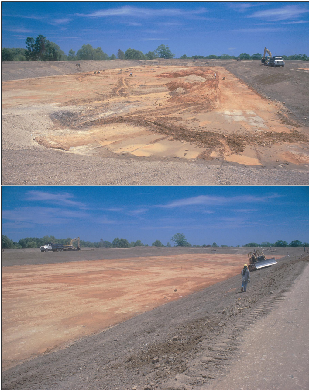
Figure 9.5 Impermeabilization of ponds with clay which is essential to maintain the water balance and avoid excessive infiltration, with the possible contamination of the groundwater. The clay should be layered with a total thickness of at least 5–10 cm, and covered with a layer of soil to protect it. In this example, the contractor did not put clay on the interior slopes and the pond had excessive infiltration as seen in Figure 9.4 (La Ceiba, Honduras).
