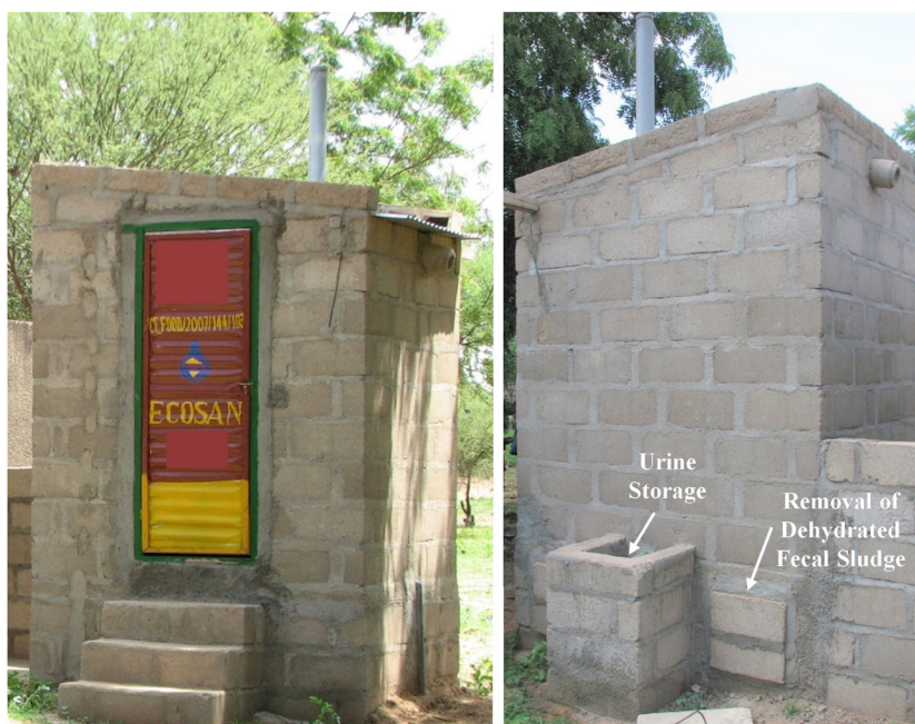
Figure 7.10 An ecosan dehydration toilet with urine diversion operated at a nongovernmental organization education center in Burkina Faso. The design has two feces collection chambers in parallel that are operated as batch reactors: one chamber is in operation, while the second, filled chamber, is closed to use. In both chambers, the fecal sludge dehydrates through natural evaporation, ventilation, and the addition of absorbent materials. To be successful, water and urine should not enter the chambers. The chambers should be designed for a minimum sludge retention time of 1 year in the batch mode (WHO, 2006). Figure 7.11 shows the interior of the toilet.
