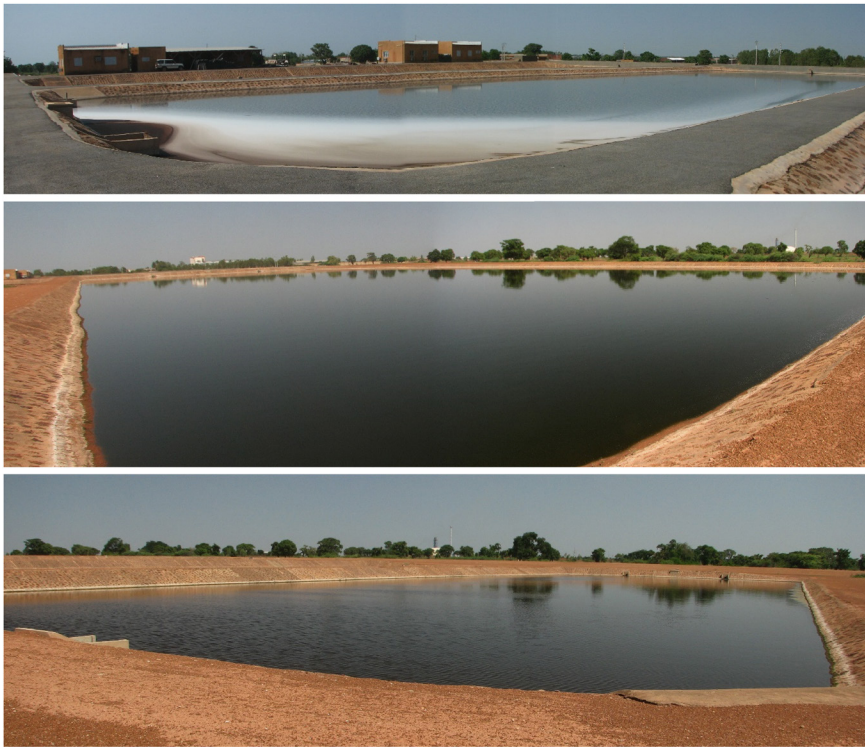
Figure 7.15 The Ouagadougou stabilization pond system. Top photo: One of the anaerobic ponds, which have historically been underloaded as a result of a low number of sewer connections. Middle photo: One of the two facultative ponds in operation. Bottom photo: Maturation pond 3, which discharges into the irrigation canal. The anaerobic ponds should be covered for methane capture.
