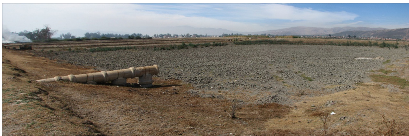
Figure 1.28 An abandoned facultative pond at the Albarrancho wastewater treatment facility in the city of Cochabamba, Bolivia. The original waste stabilization pond system built in the 1980s was designed for agricultural reuse and discharge. The growth of the city and lack of pond desludging overloaded the system in the 1990s, and a new treatment system using UASBs with trickling filters is planned. The final effluent of the new plant will discharge to the contaminated Rio Rocha. No integrated reuse in agriculture is planned, although downstream farmers could have better quality water for irrigation if the final effluent of the new plant was used directly for irrigation.
