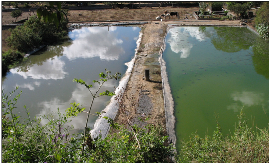
Figure 7.24 The waste stabilization pond system at Aurora II consists of a facultative pond (left) followed by a maturation pond (right). The system would produce a high-quality effluent in terms of pathogen reduction for irrigation of the cattle fodder.
