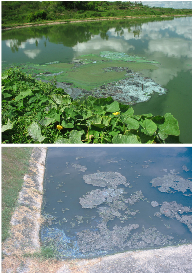
Figure 10.3 Scum, floating solids, and aquatic plants usually accumulate in the corners of ponds, driven by winds. An operator needs a scum rake and a wheelbarrow to remove these solids. If the solids are not removed frequently, they will emit odors due to decomposition and serve as suitable foci for the attraction and reproduction of insects (top photo: Lagartos, Brazil; bottom photo: Villanueva, Honduras).
