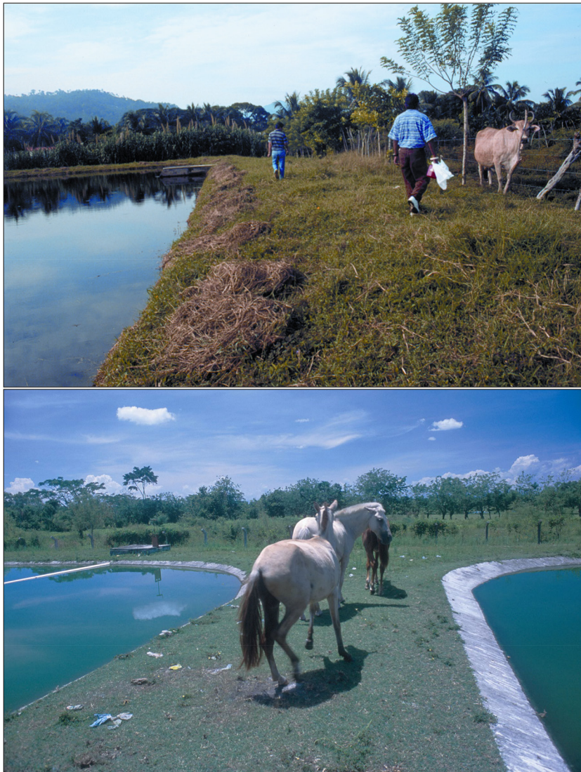
Figure 9.30 The area encompassing the entire stabilization pond system should be fenced, preferably with barbed wire, to prevent the entry of animals, which can damage embankment slopes and serve as sources of infection, and that of unauthorized persons (photo above: Tela, Honduras; photo below: Choloma, Honduras).
