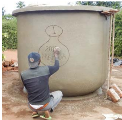
Figure 18.6 Finishing the outside. (Source: Author's own).
