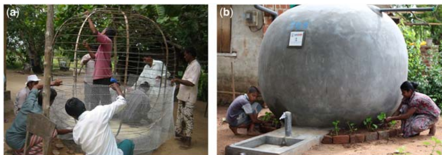
Figure 3.7 (a) Constructing a ferrocement pumpkin tank. (Source: LRWHF, s.f). (b) Finished ferrocement pumpkin tank. (Source: LRWHF, s.f).
