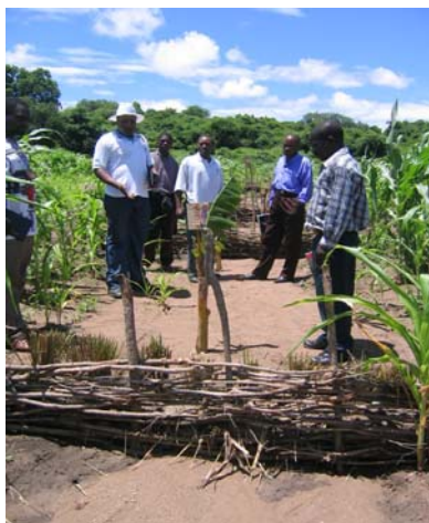
Figure 11.13 Check-dams, Karonga District. (Source: Author's own).
