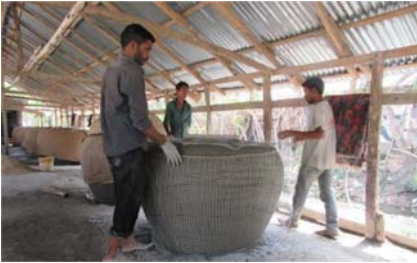
Figure 7.7 Reinforcement with wire net. (Source: Author's own).
