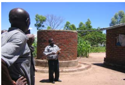
Figure 11.2 Above ground brick tank, Karonga District. (Source: Author's own).
