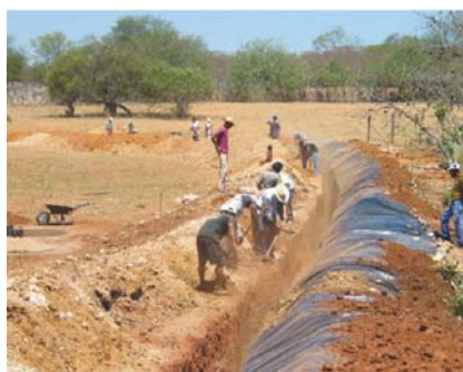
Figure 16.7 Sub-surface dam construction, placing the PVC sheet. (Source: Author).
