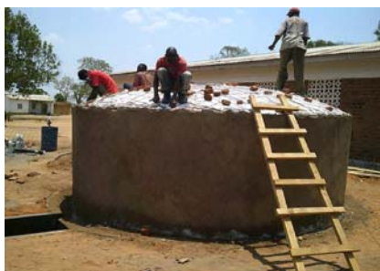
Figure 11.5 Ferro-cement tank under construction. (Source: Author's own).
