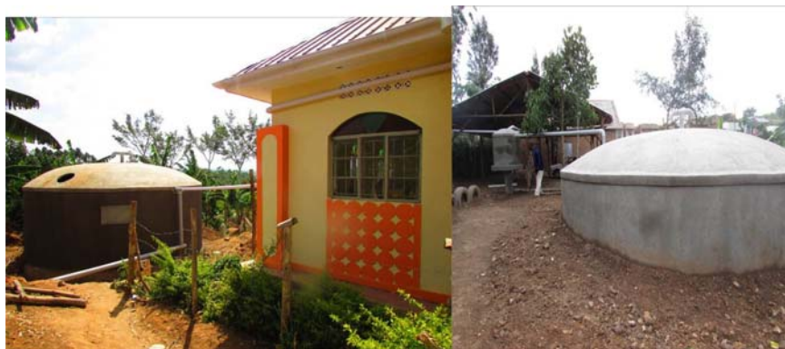
Figure 9.1 50 m 3 ferrocement tanks. (Source: Kikundwa Anne).
