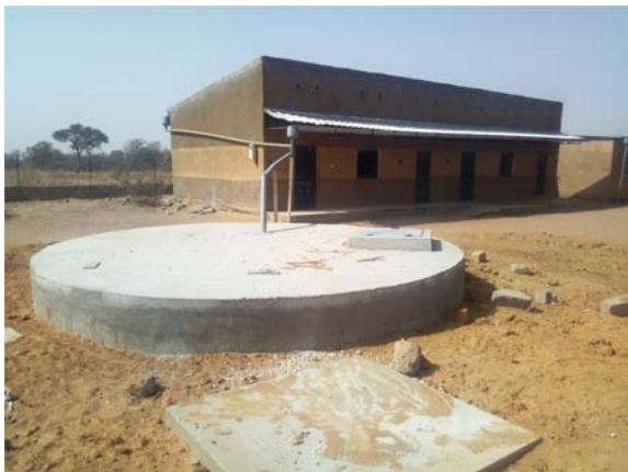
Figure 10.2 Rainwater harvesting system in Dekhaye School. (S.Sene, 2018).
