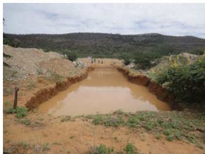
Figure 16.5 A four-meter deep trench-like rock cistern stores water for goats. (Source: Author).
