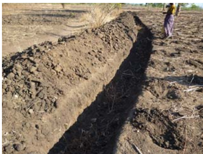
Figure 11.11 Infiltration pit, Neno District. (Source: Author's own).
