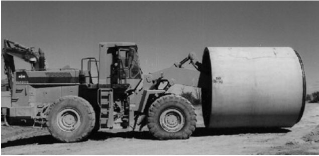
Figure 14-3. Special equipment to handle a large concrete pipe.
