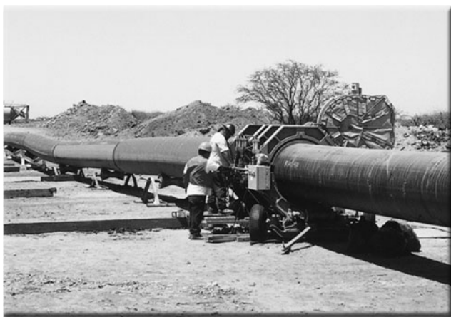
Figure 18-3. Joining HDPE pipe by heat fusion. Reprinted with permission from Performance Pipe, Plano, TX.
