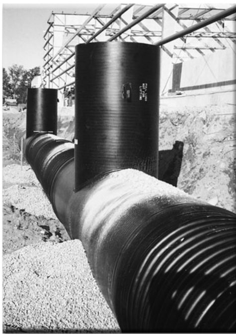
Figure 18-2. HDPE pipe with ASTM F 894 profile walls, bell-and-spigot jointed. Reprinted with permission from Performance Pipe, Plano, TX.
