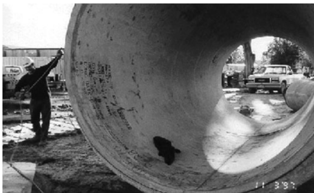
Figure 7-1. Pipe markings inside a concrete pipe. Courtesy of Price Brothers Corporation.
