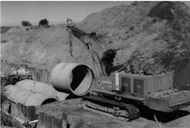
Figure 14-5. Installing large-diameter concrete pipe.
