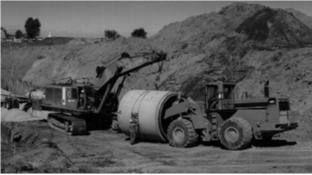
Figure 14-4. Equipment handling large concrete pipe.
