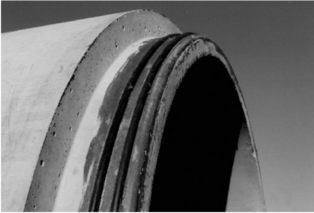
Figure 14-1. Spigot end of reinforced concrete pipe used on the sample project.
