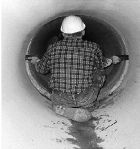
Figure 13-5. Engaging a field joint in a PCCP. With the pipe joints clean and lubricated, proper alignment of the spigot and bell allows easy engagement of the pipe ends. Courtesy of Price Brothers Corporation.
