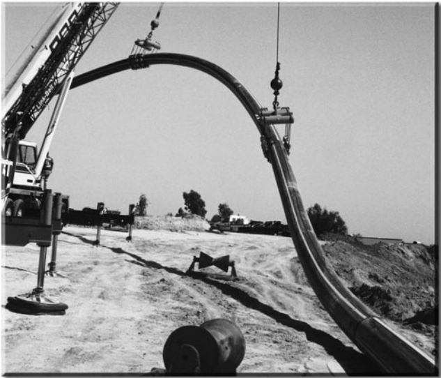
Figure 18-5. Flexibility of HDPE pipe eases installation. Reprinted with permission from Performance Pipe, Plano, TX.
