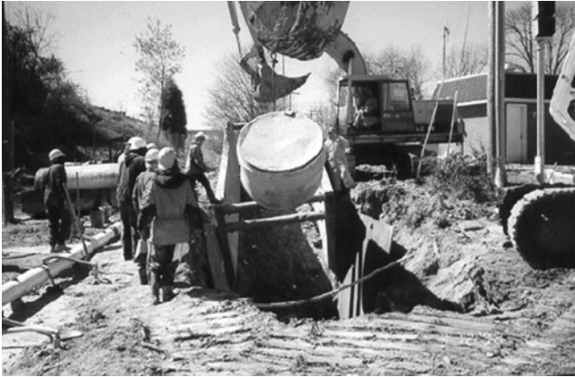
Figure 13-3. Setting a pipe and pipe bend combination. Note the end cap on the bend, the dual lifting points, the spotters, and the trench box and trench sheeting. Source: Gannett Fleming, Inc. Used with permission.
