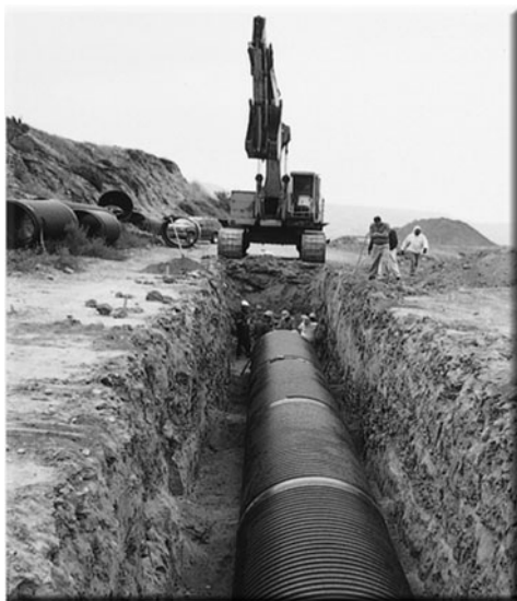
Figure 18-4. Installation of ASTM F 894 pipe for conveyance of foul air. This excavation is in a rock-hard, caliche-type soil. Reprinted with permission from Performance Pipe, Plano, TX.
