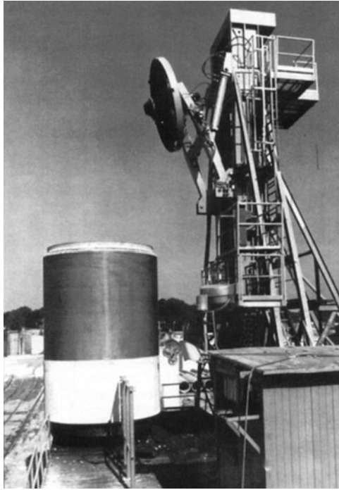
Figure 13-1. Wrapping a prestressed concrete pipe. Courtesy of Price Brothers Corporation.
