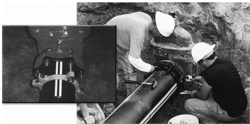
Figure 18-6. Mechanical connection of HDPE pipe to a valve. Reprinted with permission from Performance Pipe, Plano, TX.
