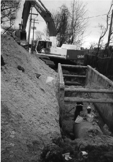
Figure 13-4. A trench box in service. Courtesy of Price Brothers Corporation.
