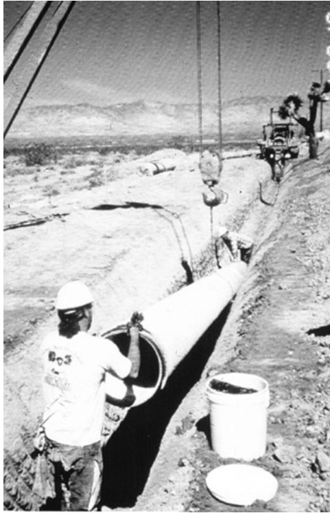
Figure 15-1. Installing a typical reach of bar-wrapped concrete cylinder pipe. Copyright © Boyle Engineering Corporation. Used with permission.
