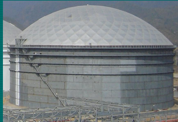
Dome Roof Tank
