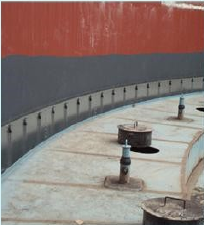
( WB-1 Pantograph Type Mechanical Shoe Seal )
