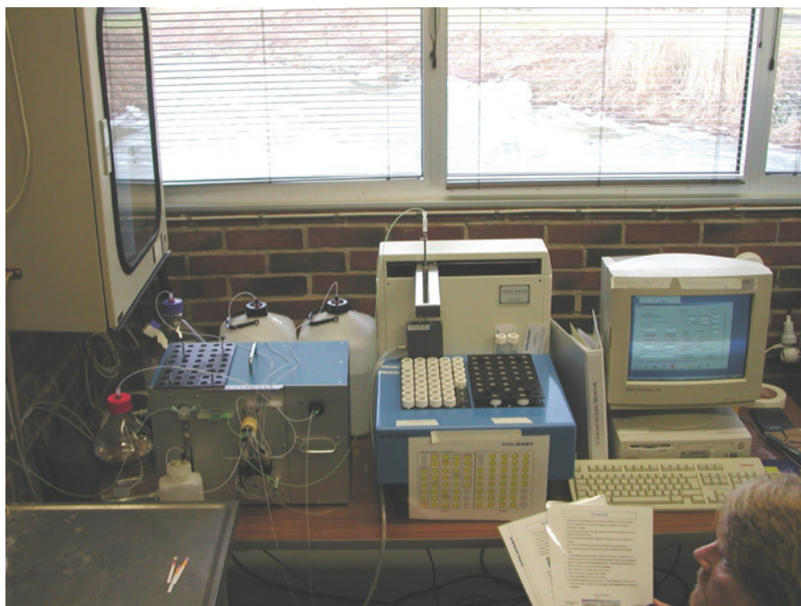
Figure 6.10 CALM model 1 installed in 2003 at the Göta river raw water intake building.
