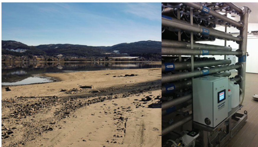
Figure 6.12 The Colifast ALARM installed at the filtration rig, Jevnaker WTP, by Lake Randsfjorden, Norway.
