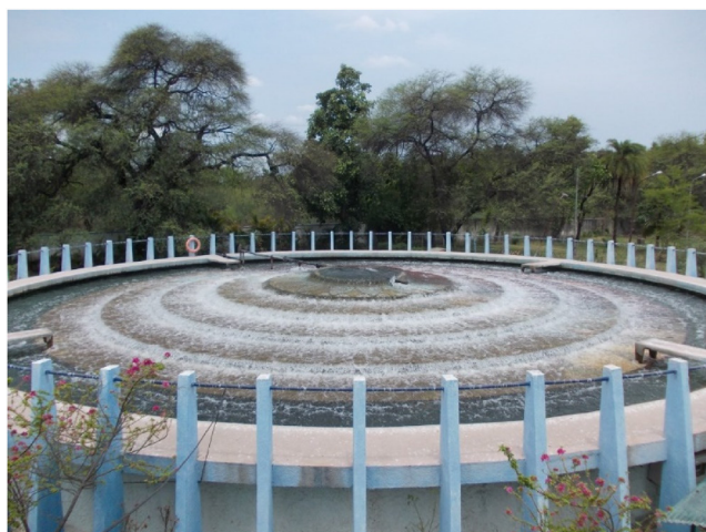
Figure 2.6 Cascade aerator in water treatment plant (courtesy of Nagpur Municipal Corporation and Orange City Water Private Limited, Nagpur, India).
