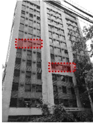
(a) Office building – rooms 01 and 02 (Northwest façade)
