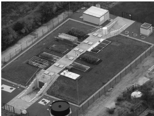
Figure 5.1.1 The pilot scale plant in Leuna (courtesy of M. Kaestner).
