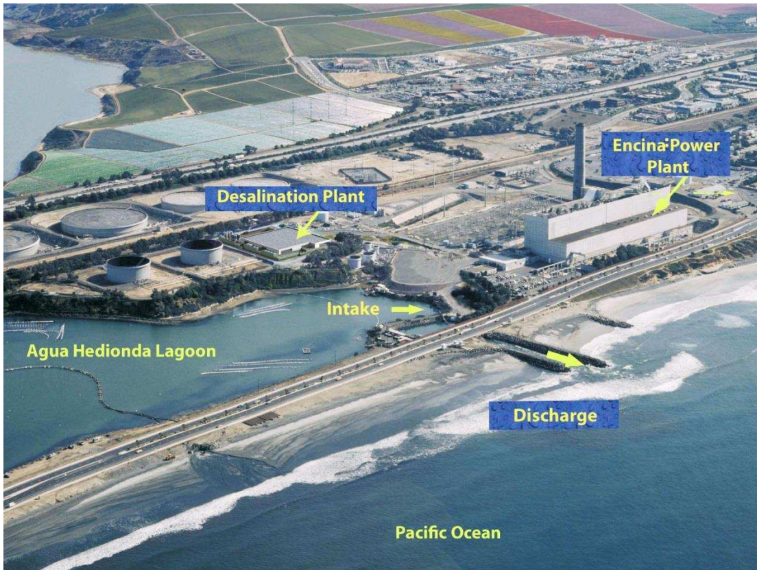
Figure 8.1. Carlsbad Desalination Plant Showing Discharge Location.
