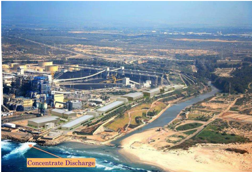
Figure 3.1. Near-shore Discharge of the Hadera SWRO Plant, Israel.
