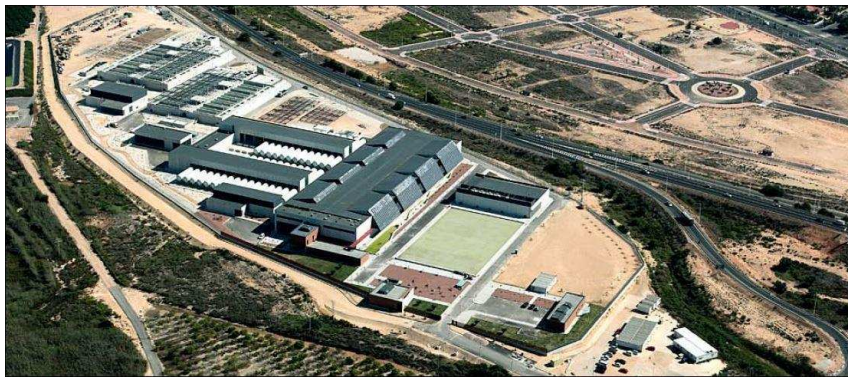
Figure 10.9. Torrevieja Desalination Plant, Alicante, Spain.
