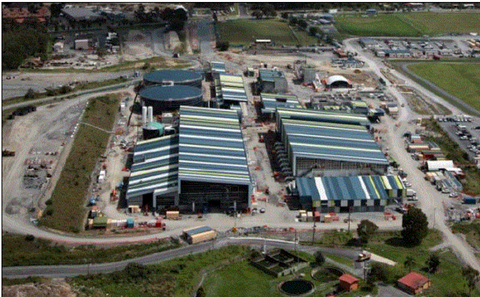
Figure 10.7. Gold Coast Seawater Desalination Plant.
