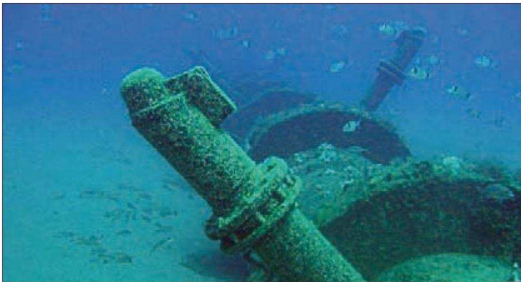
Figure 10.10. Capped Ocean Outfall Pipe.
