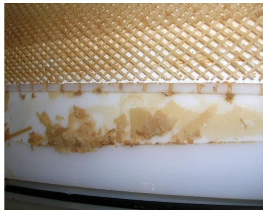
Figure 3-5: Scale formation blocking the cassette flow channels
