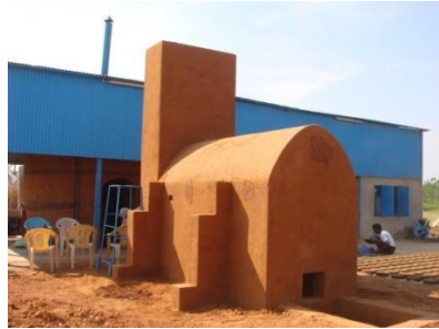
Kiln constructed for cindering discs
