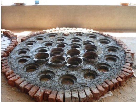
Casting of R.C.C. Terrafil Disc Holder
