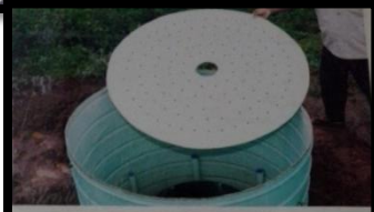
3. Placing filter plate
