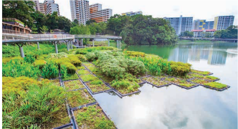
Fig. 10.32 Floating wetlands, a type of ABC Waters design feature, filter and cleanse water naturally without the use of chemicals
