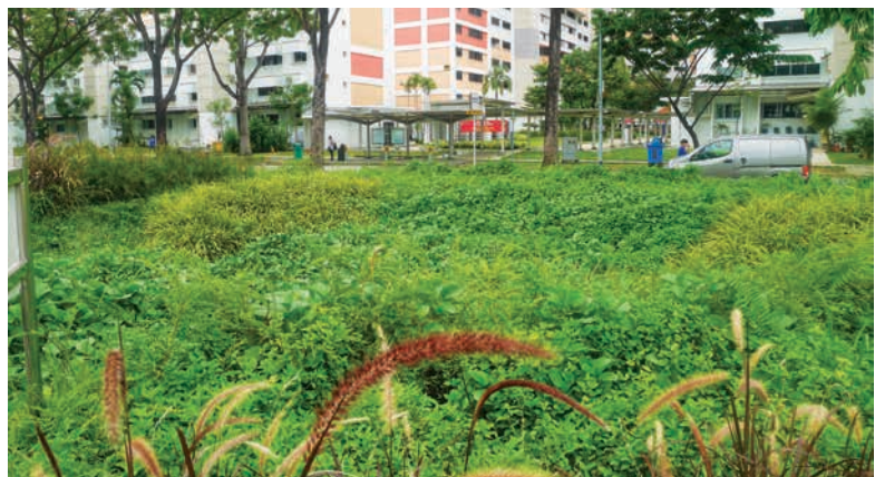
Fig. 10.9 Rain garden treats runoff from adjacent road and plaza space
