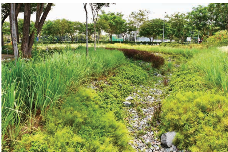
Fig. 10.42 Bioretention swales and vegetated swales help to slow down and cleanse rainwater runoff before discharging to Kallang Basin and Marina Reservoir
