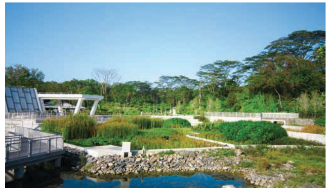
Fig. 4.4 Cleansing biotopes installed at the Central Plaza in Jurong Eco-Garden
