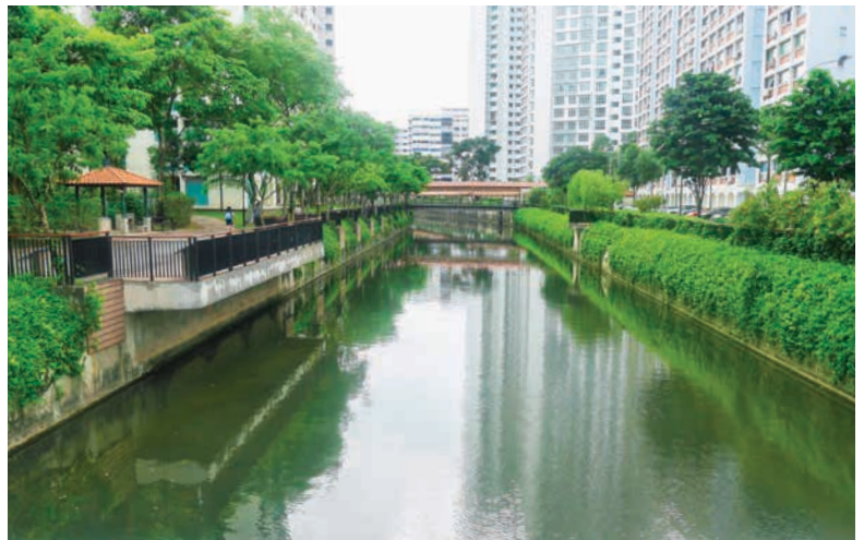
Fig. 4.46 Greening of canal wall at Sg Whampoa-St George's Lane
