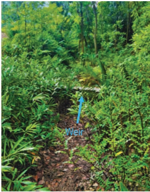
Fig. 10.21 Along the vegetated swale at the outlet of the Canarium pond, a weir (a barrier across the horizontal width of the swale) was constructed
