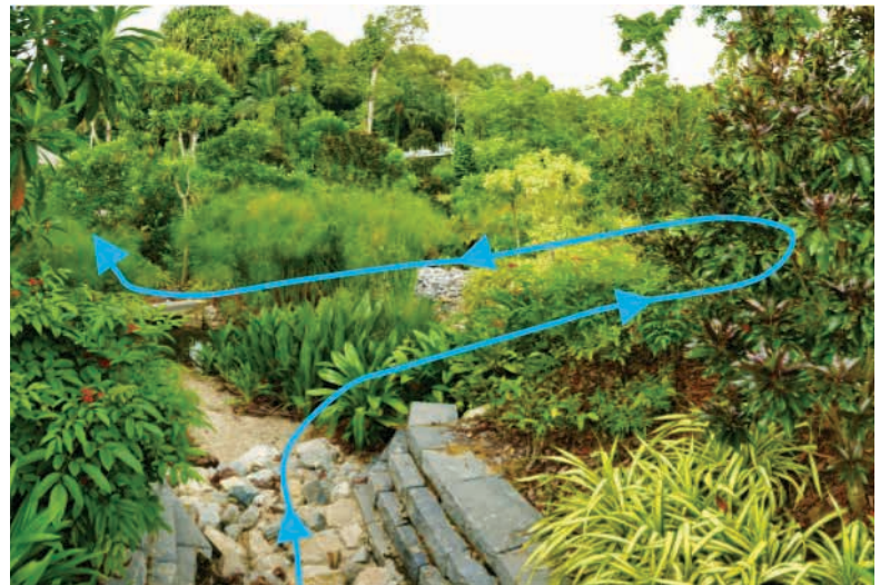
Fig. 10.23 The Cerbera Pond is a sedimentation basin that collects runoff from more than 2-hectares of land, including the coach park and carpark. A curve in the pond increases the length of the conveyance path, which promotes higher rates of detention, sedimentation and infiltration. The dense vegetation along the path enhances the biological removal of excess nutrients from the water.
