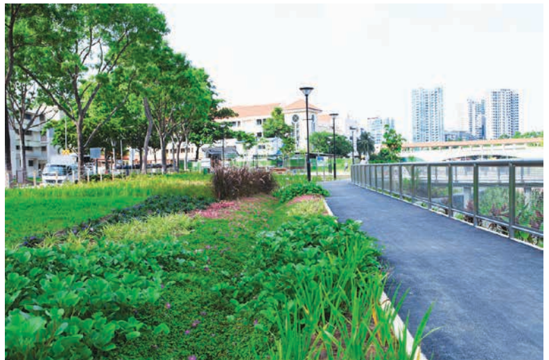
Fig. 4.27 Bioretention swale along Kallang River at Potong Pasir
