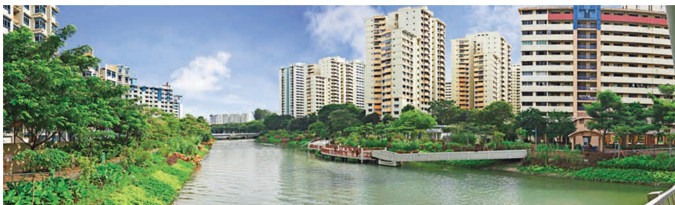
Fig. 1.4 Kolam Ayer ABC Waterfront – Floating deck to bring communities closer to the waterbody
