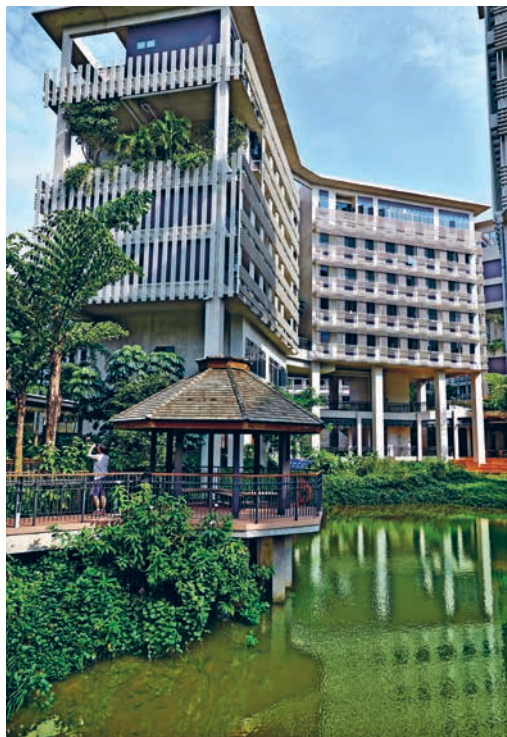
Fig. 10.27 Pioneer and Crescent Halls, set amidst lush greenery, waterscape and outdoor community spaces
