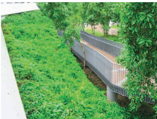
Fig. 10.57 Rain gardens are seamlessly integrated within both precincts as part of the landscape, yet provide treatment of runoff received at the e-decks
