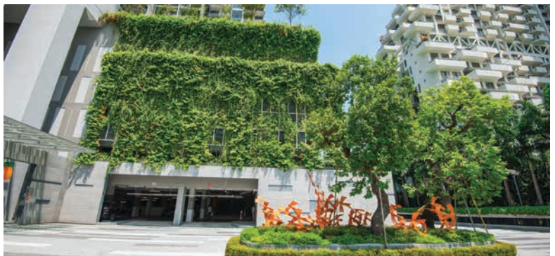
Fig. 10.50 Green façade incorporated at the entrance of the multi-storey carpark
