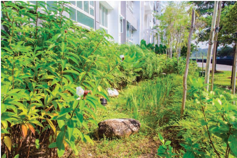
Fig. 1.6 A bioretention basin in Waterway Ridges which detains and treat stormwater runoff before discharging to downstream waterways
