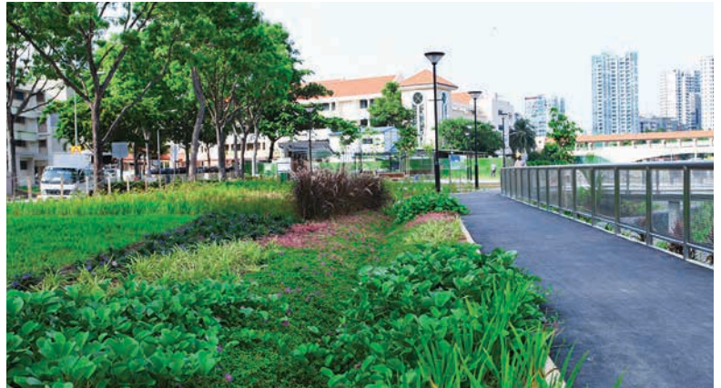
Fig. 10.10 Bioretention swales along footpath
