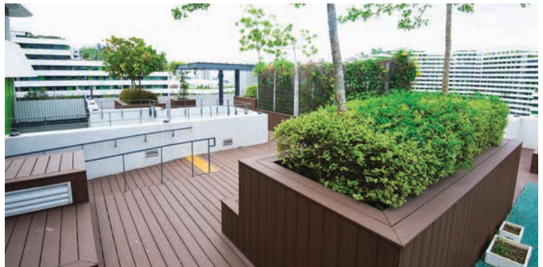
Fig. 10.58 Cascading roof gardens, made up of both intensive and extensive types of green roof, offer communal spaces for residents to gather
