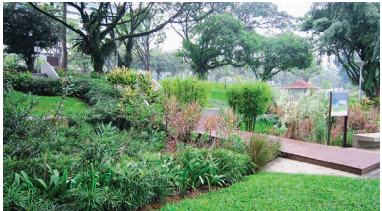
Fig. 4.32 Bioretention basin at Lower Seletar Reservoir Park
