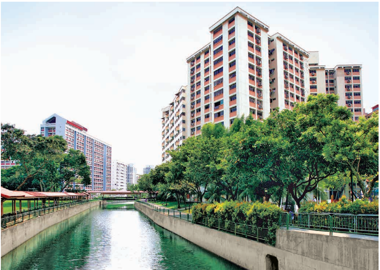
Fig. 2.1 Typical outlet drain (lined with concrete), an example of traditional stormwater management element
