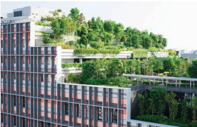
Fig. 4.12 Exterior façade of Kampung Admiralty with multi-functional greeneries
