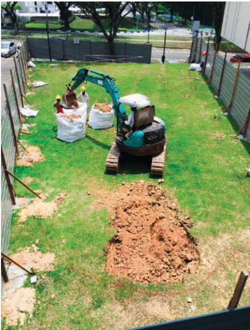
Fig. 5.1 Site is first marked out, followed by excavation
