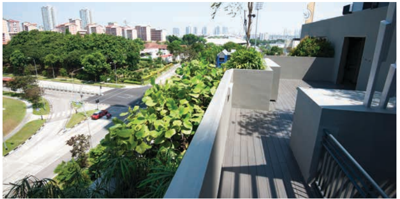
Fig. 10.49 Rain garden (planter) located on 7 th storey
