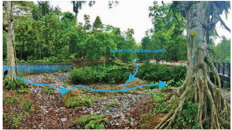
Fig. 10.22 The Canarium Pond is lined with a layer of hard rock and has been planted with plant species that are tolerant of waterlogged soils. A weir at the outlet (leading to the wetlands) of the Canarium Pond increases the pond's retention capacity and its rates of sedimentation.
