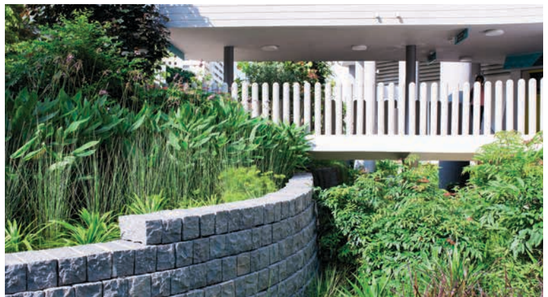
Fig. 10.15 A cleansing biotope provides natural treatment of runoff pumped up from the eco-pond
