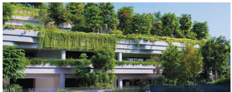
Fig. 10.13 Planters located on levels 6 (left), 7 and 8 (right) form a tiered bioretention system that provides treatment of surface runoff coming from the green roof
