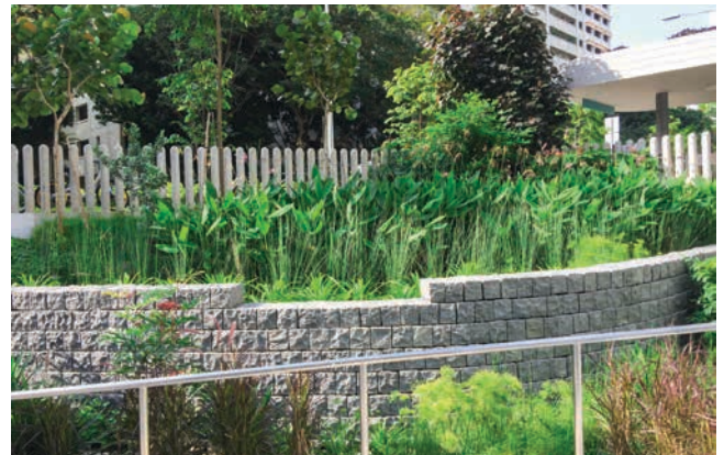
Fig. 4.13 Cleansing biotope, an ABC Waters design feature, located at ground level helps to cleanse runoff
