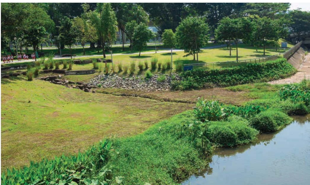
Fig. 4.48 Soil bioengineering along Kallang River @ Bishan–Ang Mo Kio Park and riparian zone along the permanent flow channel
