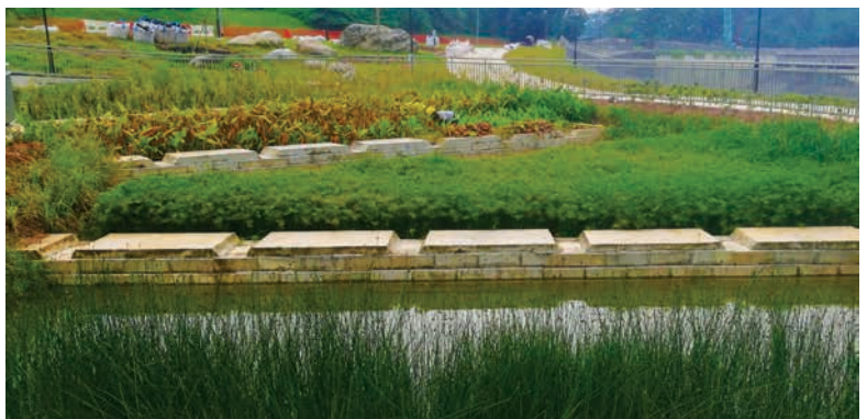
Fig. 10.3 Surface flow constructed wetland at Holland Green Node
