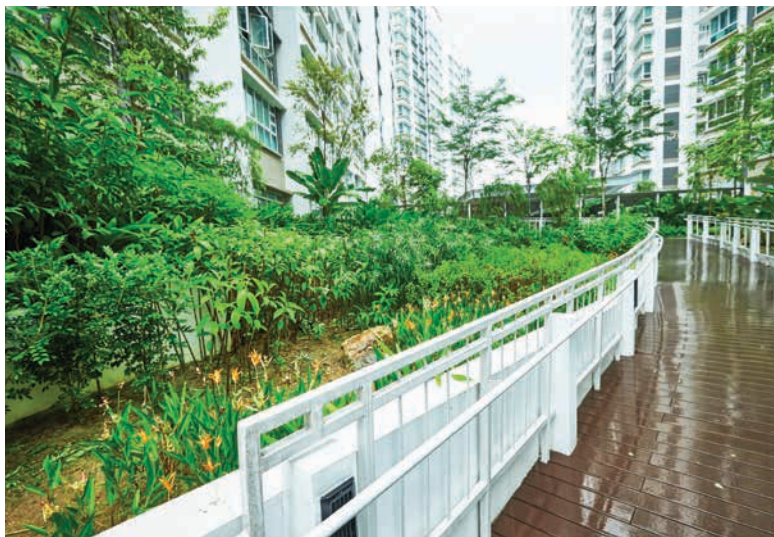
Fig. 10.52 Rain gardens are integrated within the housing precinct to enhance the aesthetics and also detains and treats rainwater runoff at the same time
