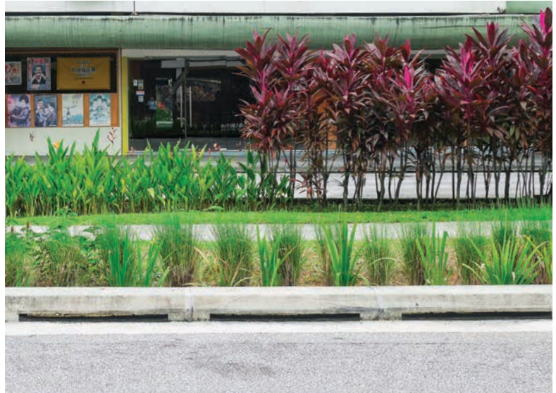
Fig. 4.14 Bioretention swale along a road with standard kerbs (with slots) in Faber Hills Estate
