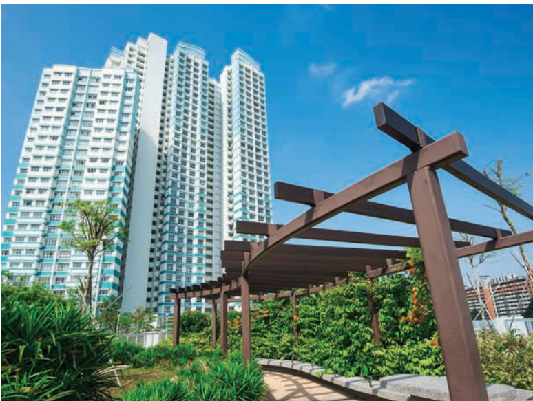
Fig. 4.6 Intensive green roof at a multi-storey carpark in Whampoa Dew
