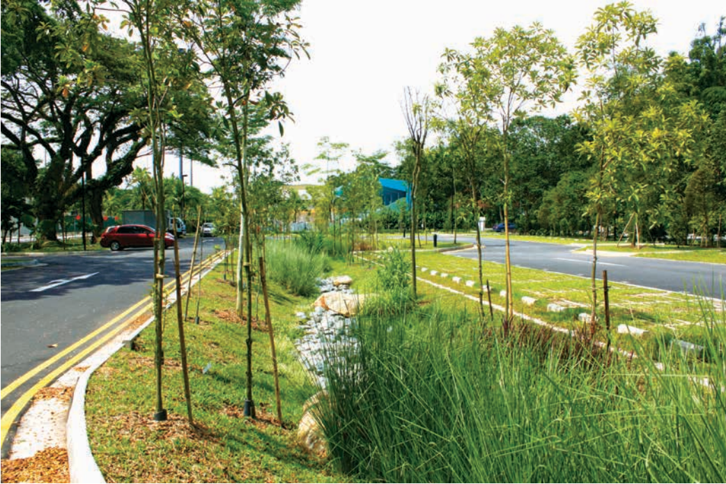
Fig. 4.21 Carpark at the Singapore Botanic Gardens with a vegetated swale to treat carpark runoff
