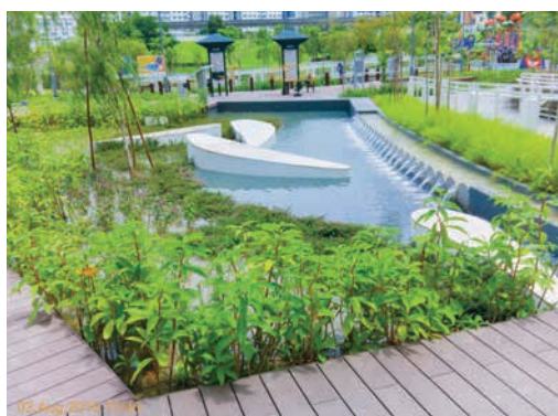
Fig. 10.54 A rain garden to showcase the cleansed water
