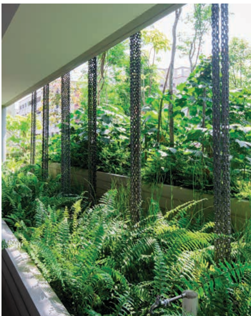
Fig. 10.13 Planters located on levels 6 (left), 7 and 8 (right) form a tiered bioretention system that provides treatment of surface runoff coming from the green roof
