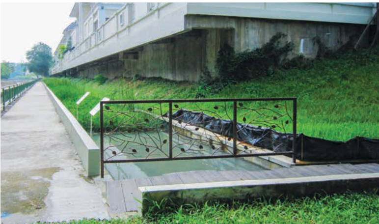
Fig. 4.36 Sedimentation forebay at Grove Drive wetland
