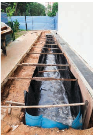
Fig. 5.2 Laying of membrane
