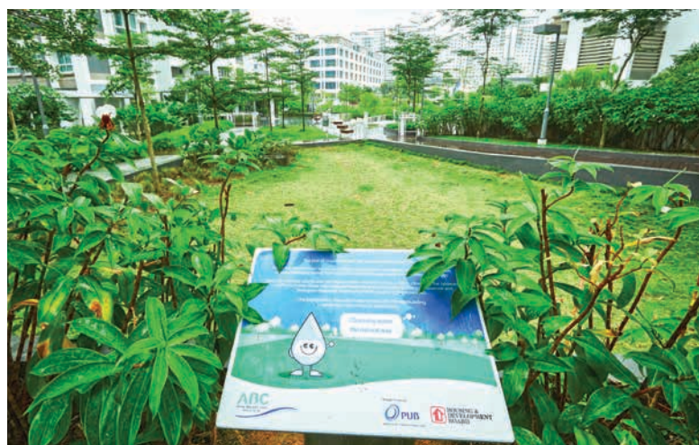
Fig. 10.55 Bioretention basin (lawn type) which doubles as a play area on dry days
