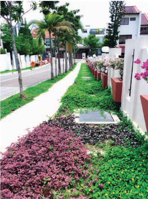
Fig. 4.22 An open concrete roadside drain along Ontario Avenue at Windsor Park Estate, Singapore has been re-configured to a lush swale with filter media to convey and clean stormwater runoff. Overflow pits are located along the swales for overflow purpose during heavy downpour, conveying excess runoff into a concrete drain beneath the swale. Low weirs are provided at suitable locations to slow down the flow of runoff.
