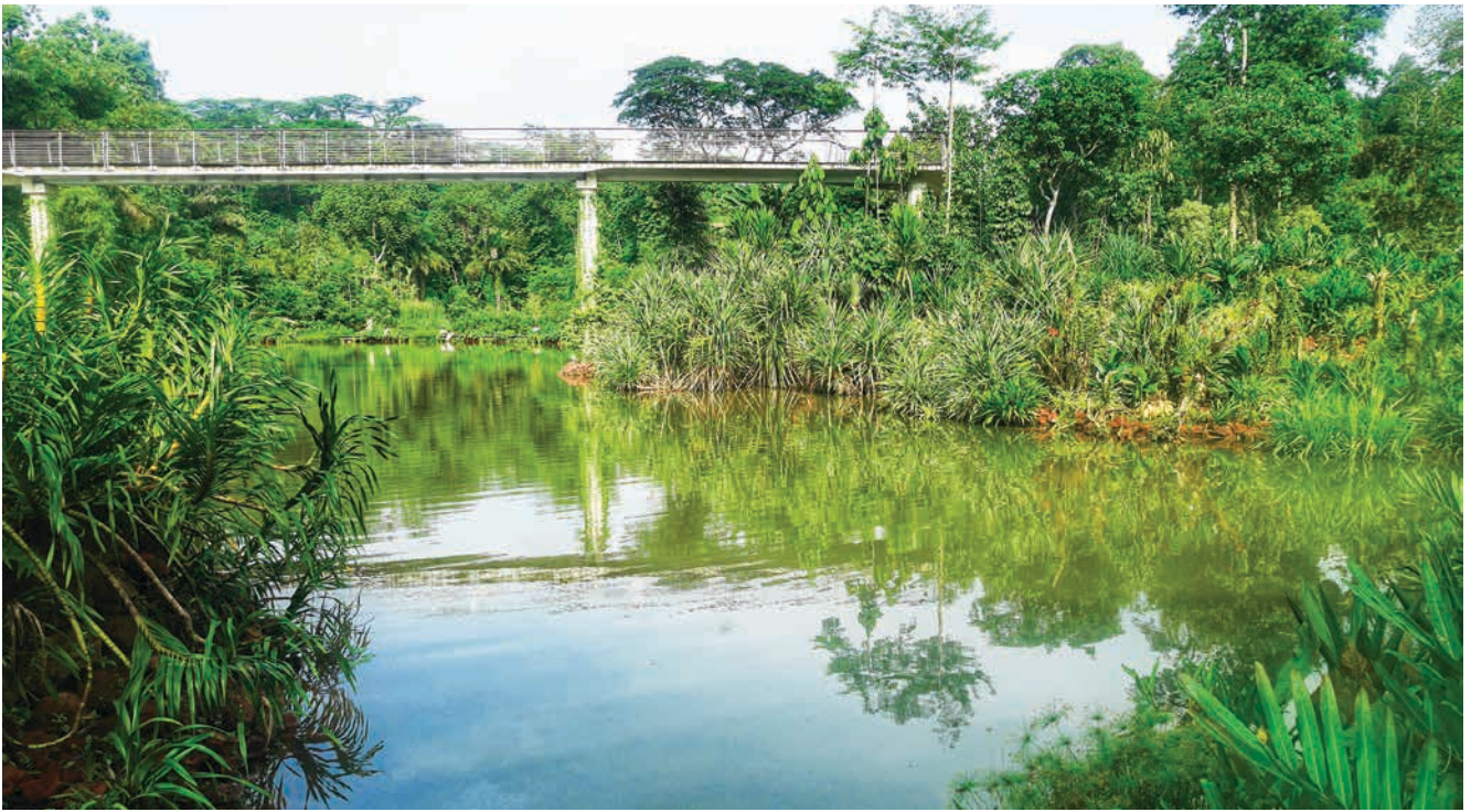
Fig. 10.24 The freshwater forest wetland removes suspended solids and the plants help to take up the excess nutrients in the water before discharging downstream to Swan Lake in the Tanglin Core of the Botanic Gardens.
