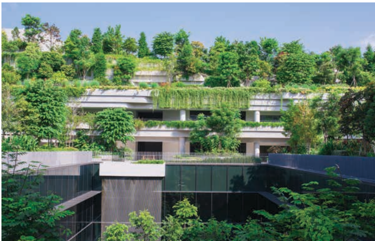
Fig. 4.5 Treatment features located at various levels of the building elements in Kampung Admiralty
