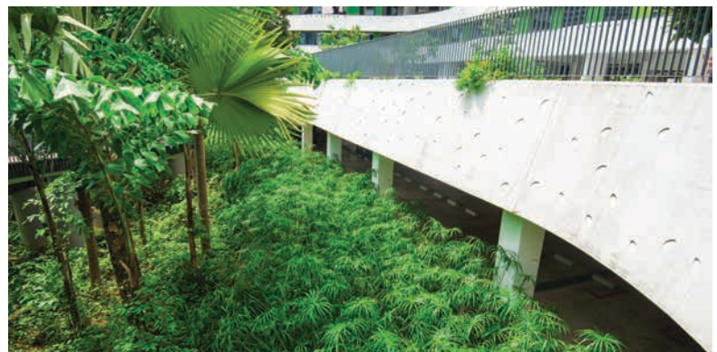
Fig. 10.57 Rain gardens are seamlessly integrated within both precincts as part of the landscape, yet provide treatment of runoff received at the e-decks
