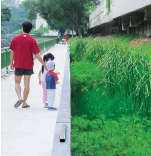
Fig. 4.38 Grove Drive surface flow wetland
