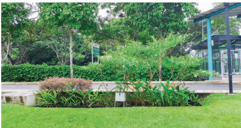
Fig. 4.29 A modular bioretention swale at NUS High School
