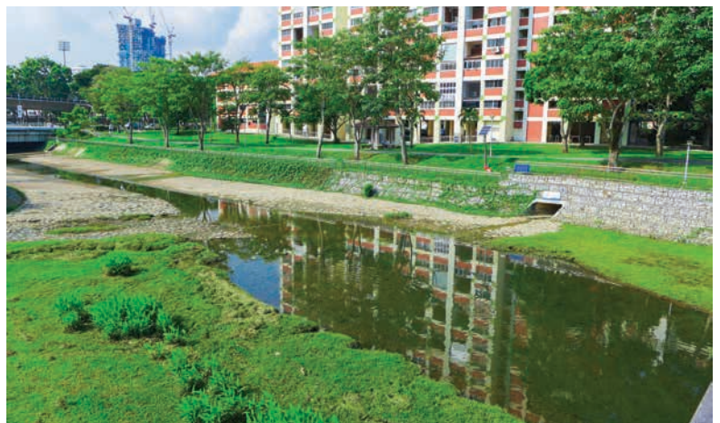
Fig. 4.47 Gabions and creepers at Kallang River @ Bishan-Ang Mo Kio Park
