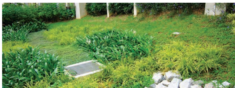
Fig. 10.29 A bioretention basin in NTU Pioneer and Crescent Halls
