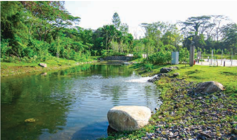
Fig. 4.35 Sedimentation basin at Jurong Eco-Garden
