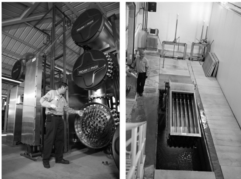
Figures 2.11 Full-scale closed vessel and open-channel UV reactors.
