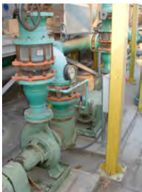
INSTALLED SUCTION DIFFUSER This is a picture of a suction diffuser installed in the field.
