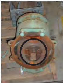
SUCTION DIFFUSER GUIDE VANES Straightening vanes (circled) ensure a uniform velocity profile into the impeller eye.
