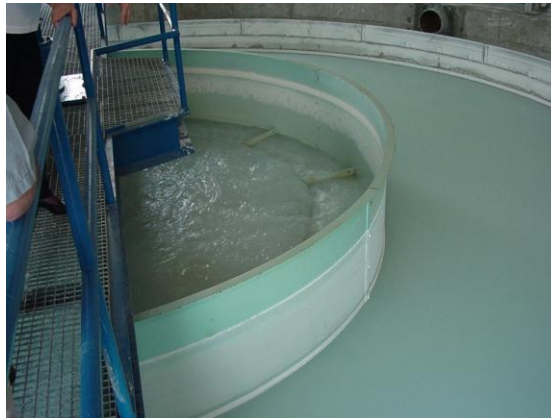
Figure 5.1: Post Treatment Lime Softening Using Slaked Lime
