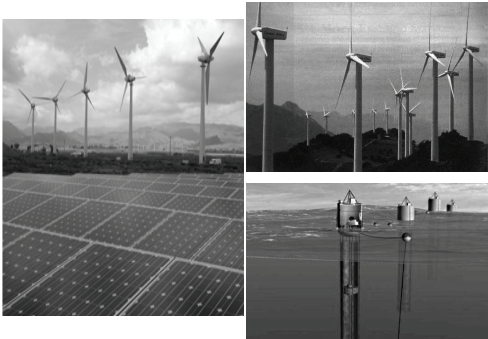
Fig. 4a (Upper Left) Wind Farm (Kalogirous, 2005); 4b (Right) Wind turbines and PV cells of Sureste SWRO plant (Sadhvani, 2008; IDA Conference, 2008); 4c (Lower Left) Wave Energy. The Aquabuoy 2.0 is a large 3 meter wide buoy tied to a 70-foot-long shaft. By bobbing up and down, the water is rushed into an acceleration tube, which in turn causes a piston to move. This moving of the piston causes a steel reinforced rubber hose to stretch, making it act as a pump. The water is then pumped into a turbine which in turn powers a generator. The electricity generated is brought to shore via a standard submarine cable. The system is modular, which means that it can be expanded as necessary (Chapa, 2007).
