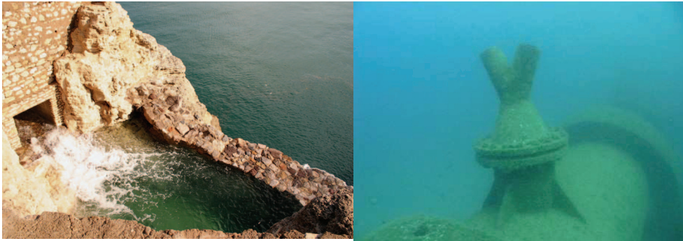
Fig. 3. Photographs of brine discharge configurations located in Spain. .A) Discharge trough a submerged outfall. B) Surface discharge .C) Discharge trough multiple jets (CEDEX).
