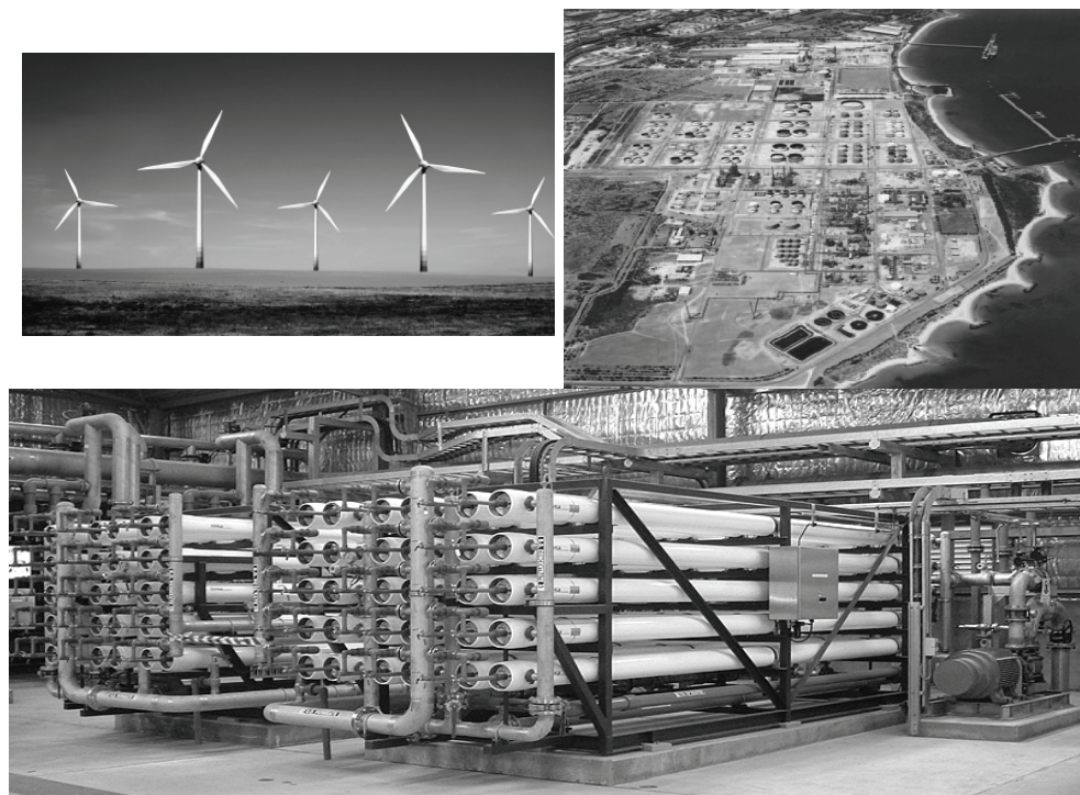
Fig. 8. The Kwinana Seawater Reverse Osmosis Desalination (SWRO) Plant and Wind Farm in Perth, Western Australia . 8a ( Upper Left ) The SWRO Plant seaside location in Pert; 8b ( Upper Right ) The Emu Downs Wind Farm consisting of 48 Vestas wind turbines each with 1.65 MW generating capacity; 8c ( Lower ) The desalination plant, with 12 SWRO trains with a capacity of 160 megalitres per day and six BWRO trains delivering a final product of 144 megalitres per day. (Pankratz, 2008).
