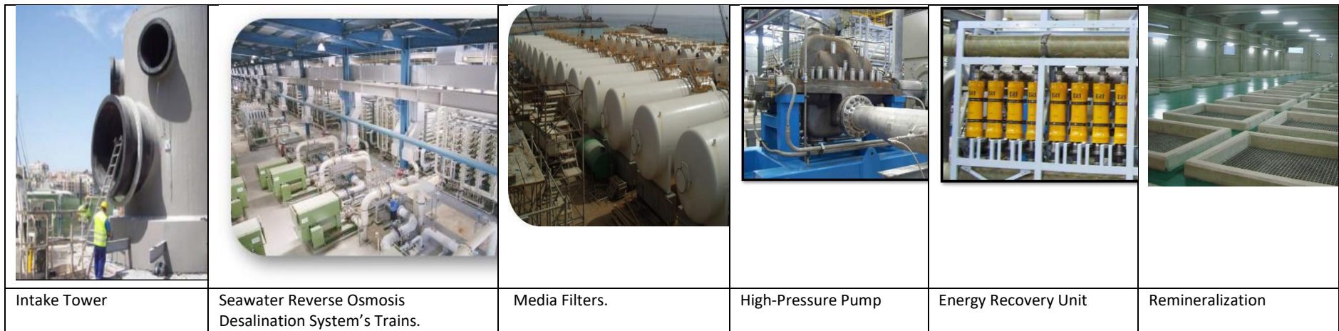
Figure 2: Typical Seawater "RO" System [SWRO]
