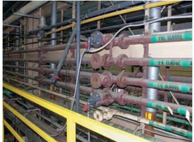
Figure 2.6 Single Pass DSS – Sampling Ports
