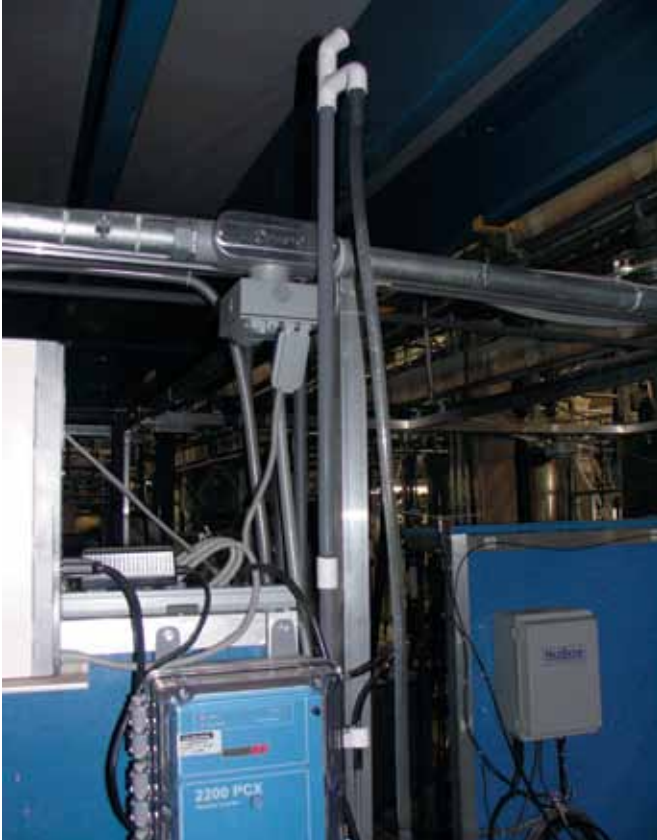
Figure 3.3 Example Constant Head Mechanism for Hach 2200 PCX Particle Counter.
