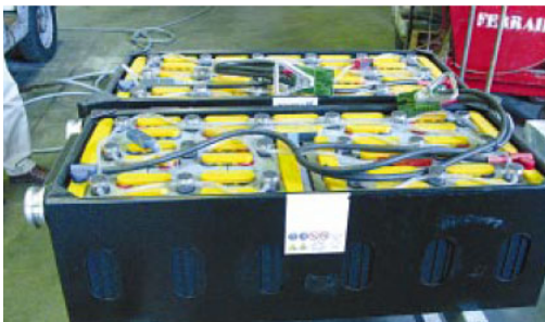
Figure 5: Set of batteries
