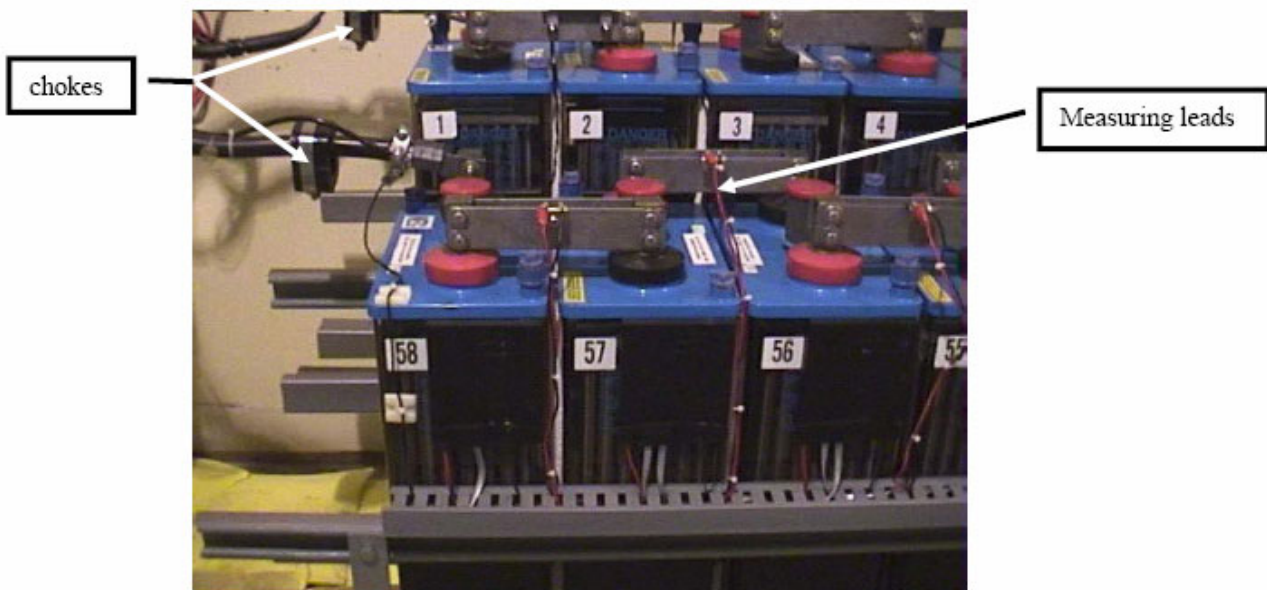
Figure 110: Installation of sensing device on each cell
