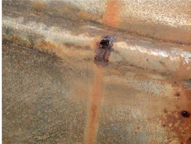
Figure 3.20 Corrosion found at a circumferential weld at the DVWTP
