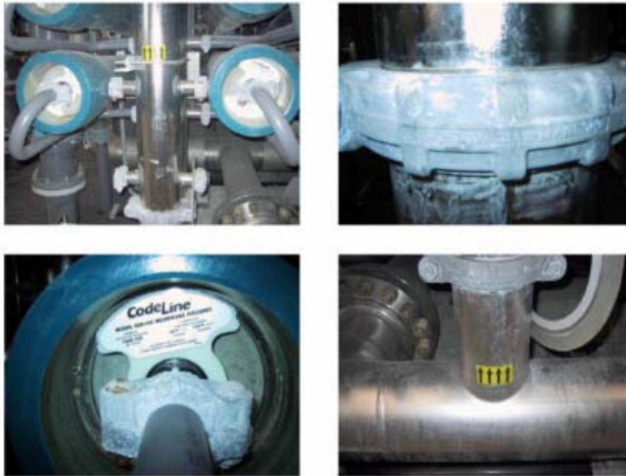
Figure 3.25 Corrosion at galvanized steel grooved couplings within the TBDP
