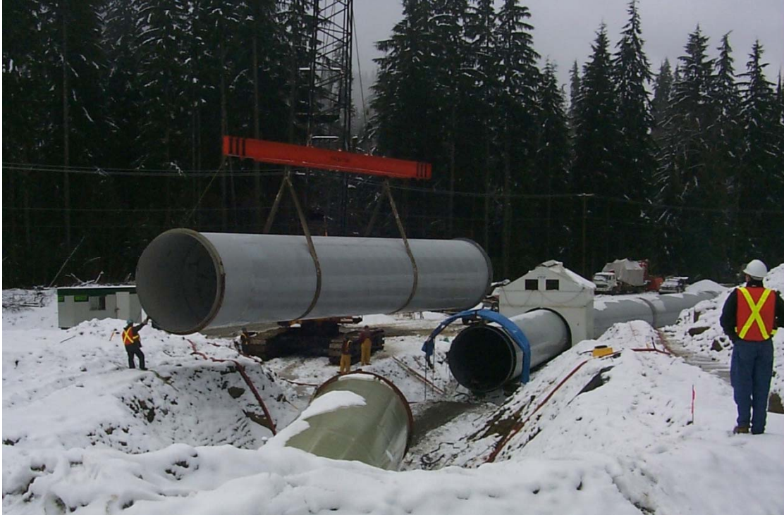
Figure 2.11 120-inch diameter stainless steel piping (Vancouver, British Columbia) made from plate material
